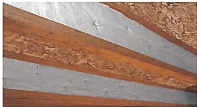
A proprietary ceramic fiber blanket insulation can be attached to the web of the I-joists to comply with IRC provisions. Photo courtesy of Mei Guo International, LLC (USA) FireBreak™.
