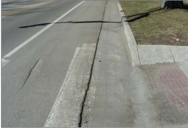
FIGURE 18: GUTTER SEAM WITHIN BIKE LANE ON WEST LAUREL STREET AT LOOMIS AVENUE
