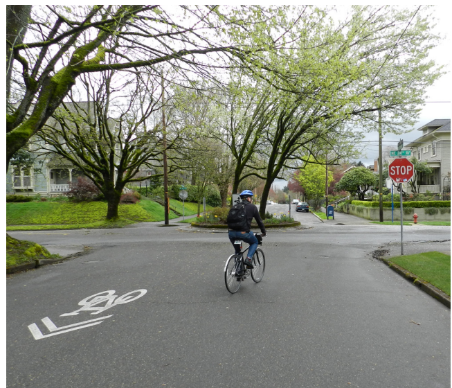
Neighborhood greenways use traffic calming such as mini circles to further slow automobile traffic
