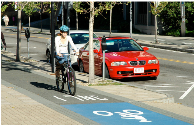
One-way, sidewalk-level, curb-separated Cambridge, Mass.
