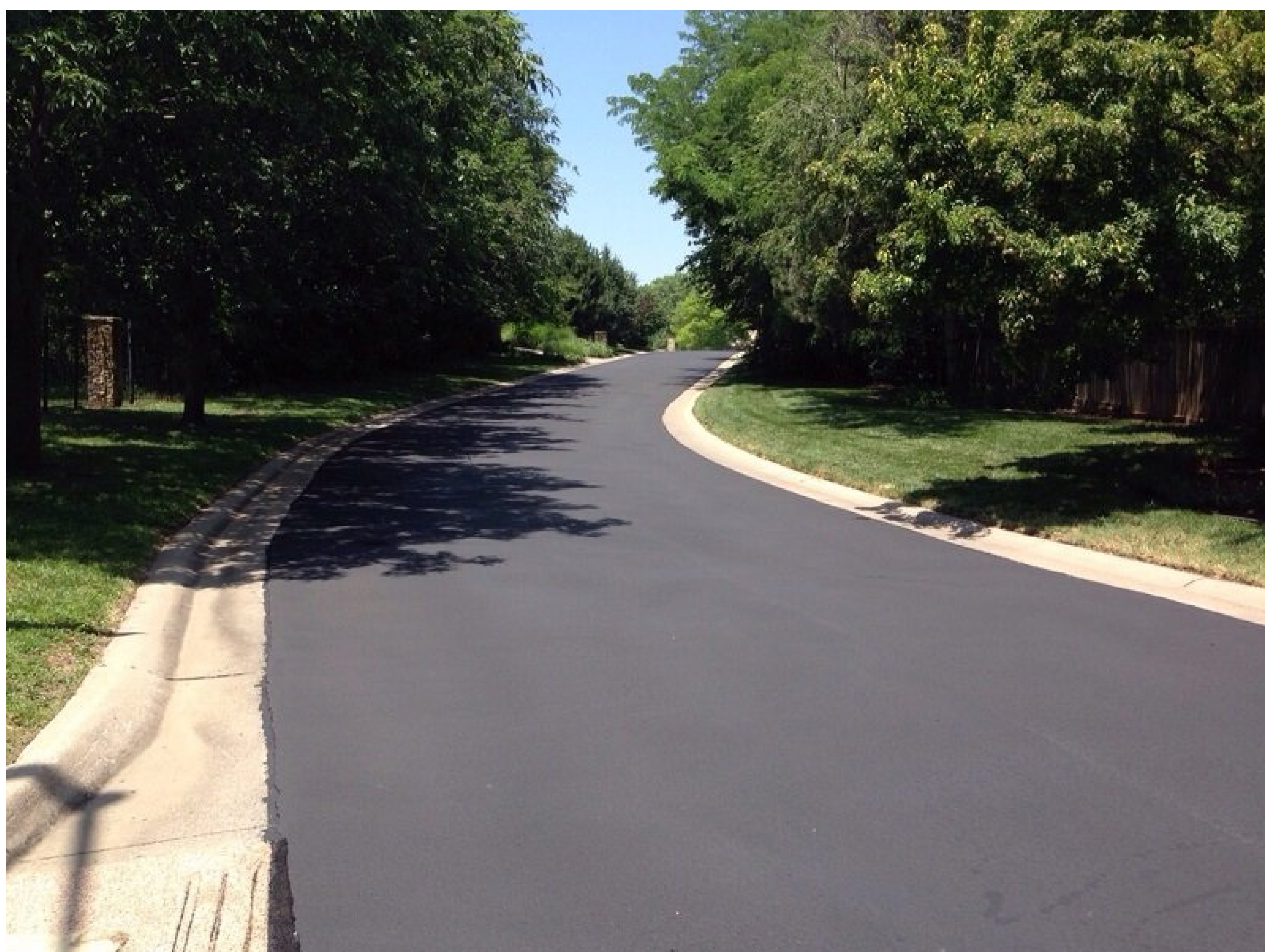
HA5 example resurfacing (Minneha, Andale Construction Inc.)
