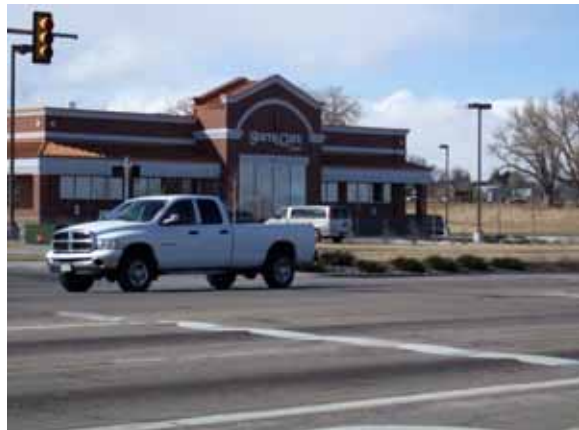
South Gate Church
