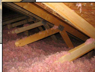
Flat attics: blown insulation Cellulose predominant, some FG
