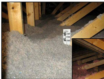
Flat attics: blown insulation Cellulose predominant, some FG
