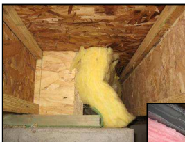
Parallel rim joists
