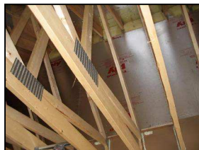
Knee walls in another 1-1/2 story Attic side fully sheathed Will perform like exterior wall Grade I
