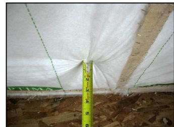
This wall blown at too low a density Grade II
