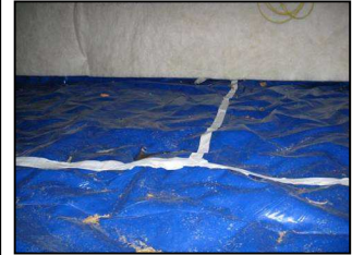
Moisture barrier details correctly handled
