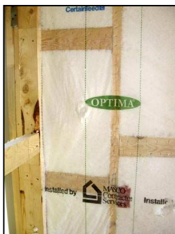
Blown FG Typically Grade I
