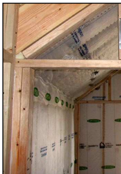
Knee walls in another 1-1/2 story Attic side fully sheathed Will perform like exterior wall Grade I
