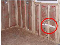
Figure 1.1.5 – Misalignment of insulation due to compression
