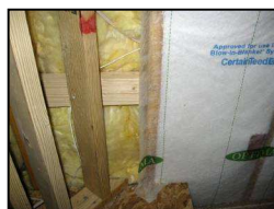
Compare batt vs blown FG at partition wall intersection
