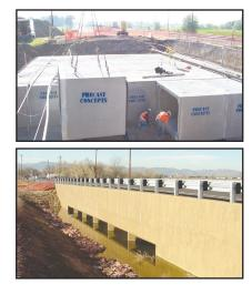
Six concrete box culverts were built and installed under East Vine Drive.
