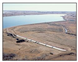
Spillway modifications at Douglas Reservoir included an erodible dam designed to release water at a controlled rate, if overtopped.
