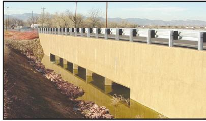
Six concrete box culverts were built and installed under East Vine Drive.
