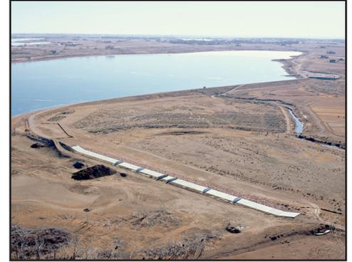
Spillway modifications at Douglas Reservoir included an erodible dam designed to release water at a controlled rate, if overtopped.
