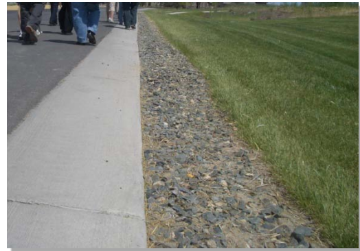
Photograph 1-2. Grass Buffer. This roadway provides sheet flow to a grass buffer. The grass buffer provides filtration, infiltration, and settling to reduce runoff pollutants.
