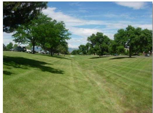
Photograph 1-3. Grass Swale. This densely vegetated drainageway is designed with channel geometry that forces the flow to be slow and shallow, facilitating sedimentation while limiting erosion.
