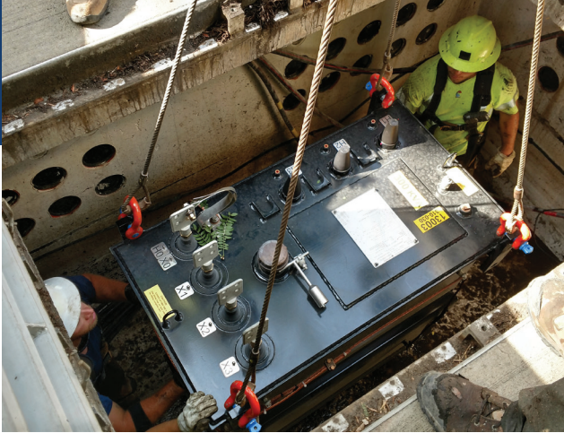
Line crews installing a new three-phase submersible transformer to maintain service reliability.
