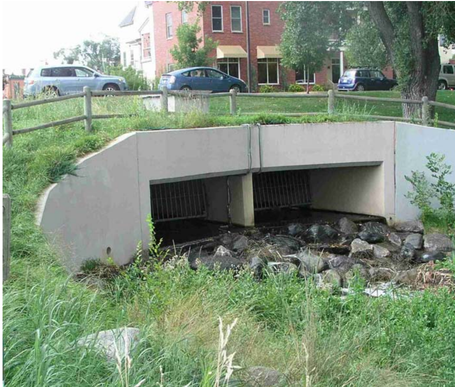
Howes Street Outfall Sampling Equipment at Lee Martinez Park
