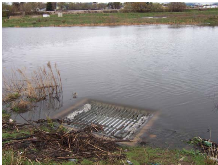
Udall Natural Area Stormwater Control Pond Outlet.
