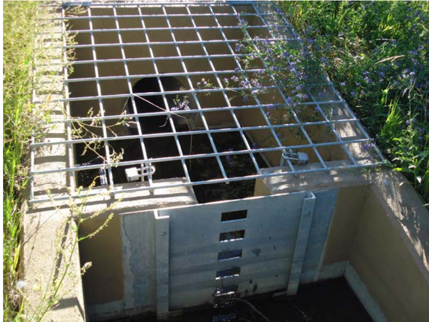
2010 Post-Construction Inspection. Note padlocks on grate.
