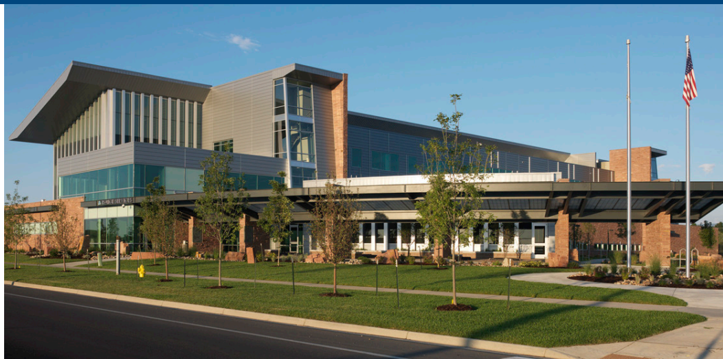
The City of Fort Collins' new Police Services Facility features daylighting, exterior spray foam insulation and evaporative condensing rooftop units.
