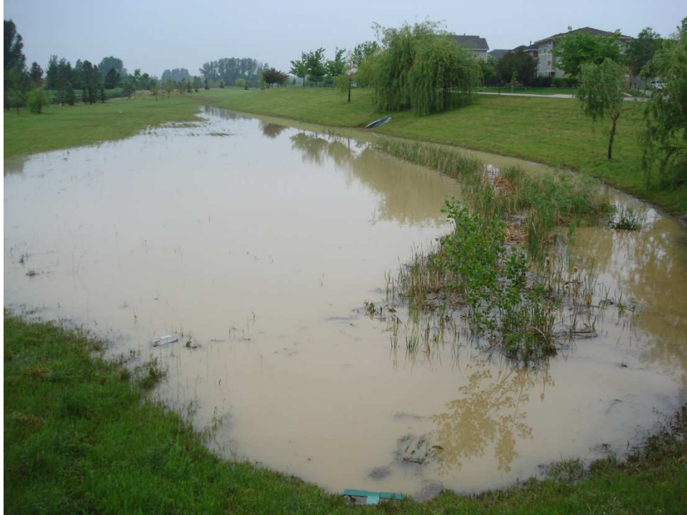
In addition to flood prevention, water quality basins are designed to detain stormwater long enough to remove sediment and associated pollutants from stormwater.
