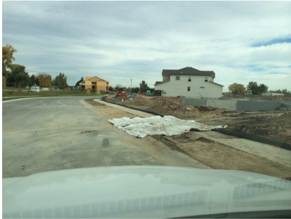
A windshield inspection reveals improper practices on this construction site, resulting in discharge of sediment to the street and gutter.
