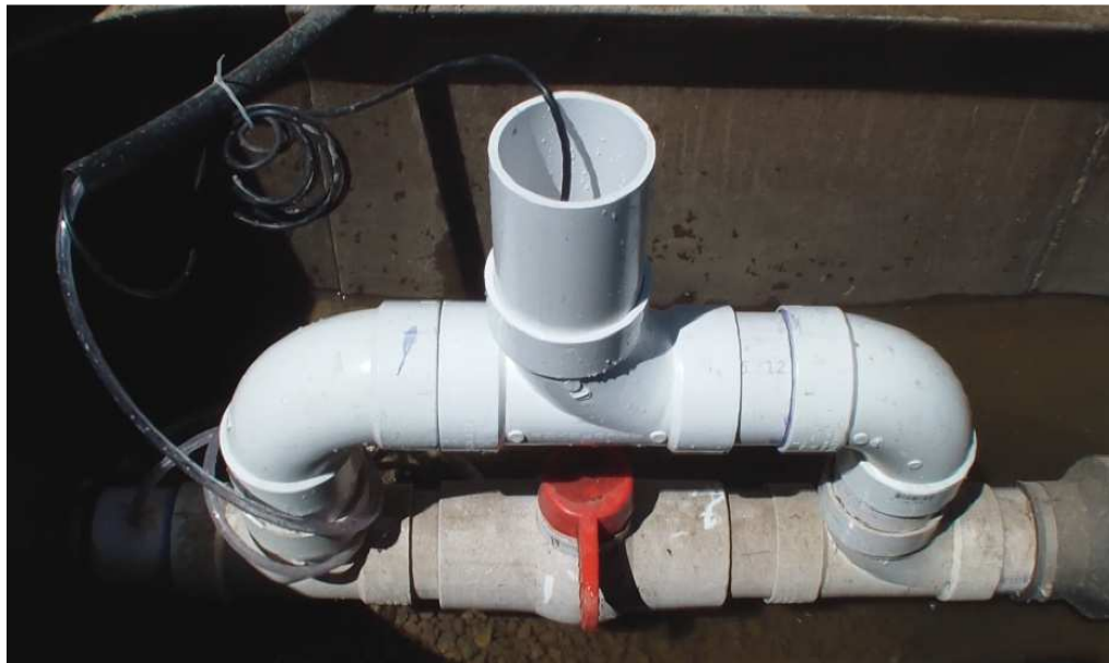
Photograph of underdrain riser configuration installed in 2014 to encourage stormwater infiltration into the ground
