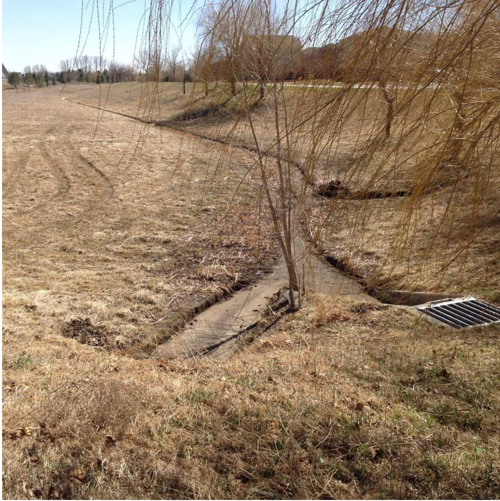
Proper maintenance of this basin entails regular cleaning of the outlet structure and removal of debris and vegetative growth from the concrete pan.
