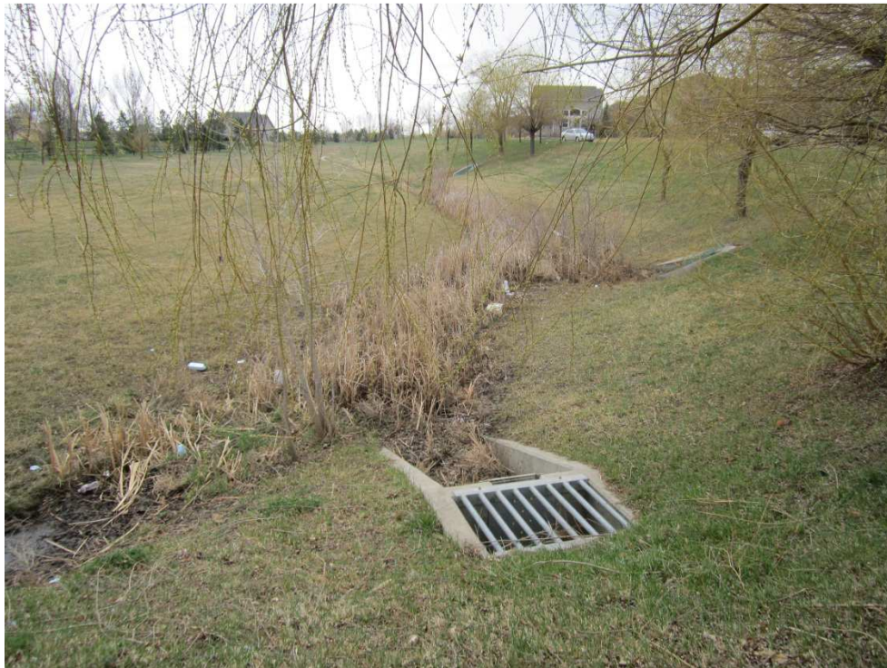
An improperly maintained water quality outlet structure can plug, causing an excess buildup of sediment and debris, and allowing excess vegetative growth in the concrete drainage pan.
