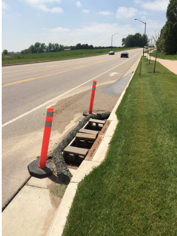
Properly installed inlet protection prevents construction site sediment and related pollutants from entering the storm sewer system inlet.
