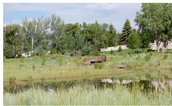
The Red Fox Meadows detention pond captures water from the west side of town and slowly releases it, minimizing damages downstream.
