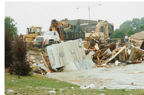
Many of the mobile homes floated off-site and became piled against the College Avenue bridge at Creekside Park.
