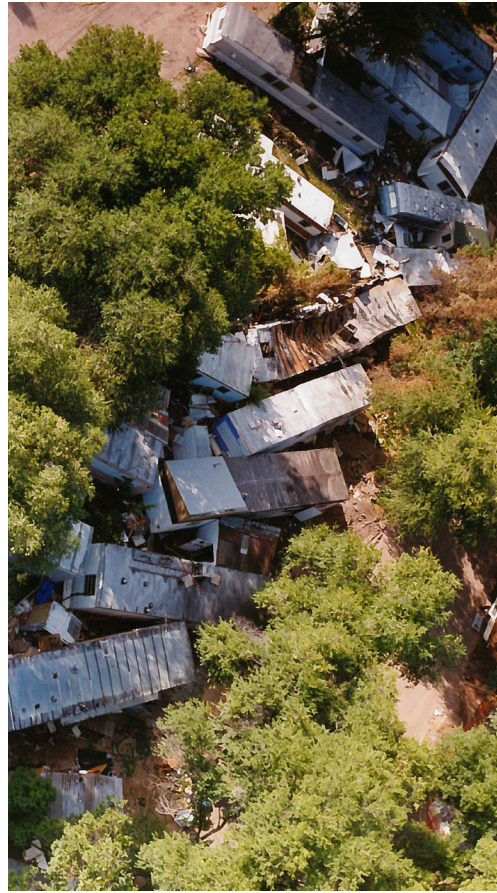
Aerial view of the Johnson Mobile Home Park showing how the mobile homes floated during the 1997 Flood.
