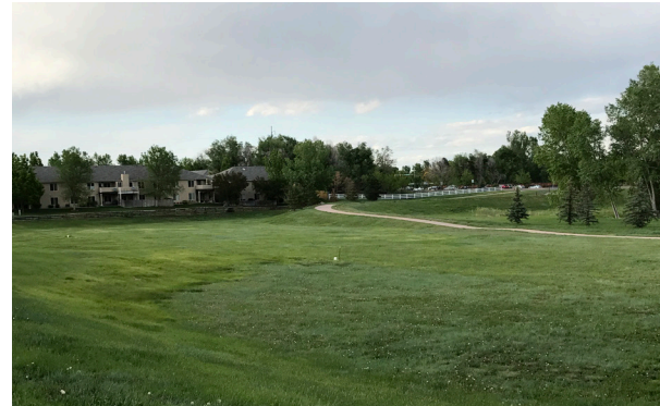
The detention pond at Taft Hill and Drake Roads was constructed after the 1997 Flood.
