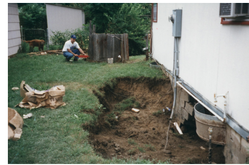
This home in Old Town had significant damage to the building foundation during the 1997 Flood.
