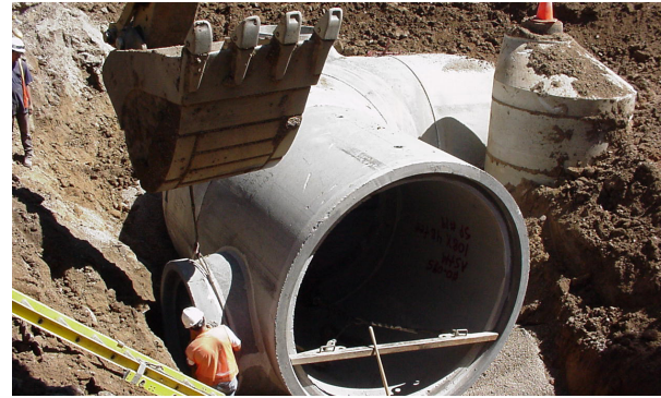
Construction of the Oak Street outfall in Old Town. These large storm sewers provide flood protection to many businesses and residences.
