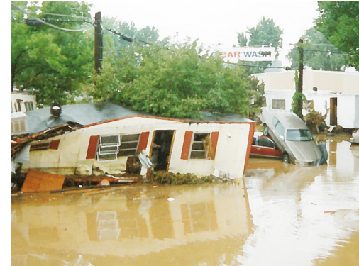
The Johnson Mobile Home Park near the Dairy Queen on South College Avenue was destroyed by the flood. There was a significant search and rescue effort that took place in this area.
