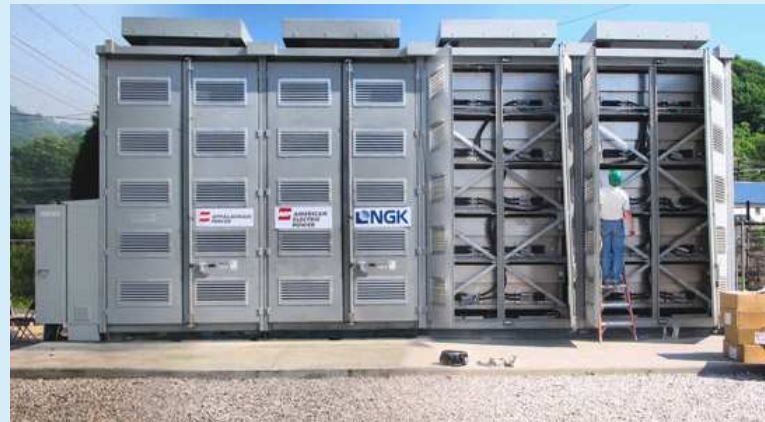
Sodium Sulfur Battery Bank (1 MW - 6 hs)
