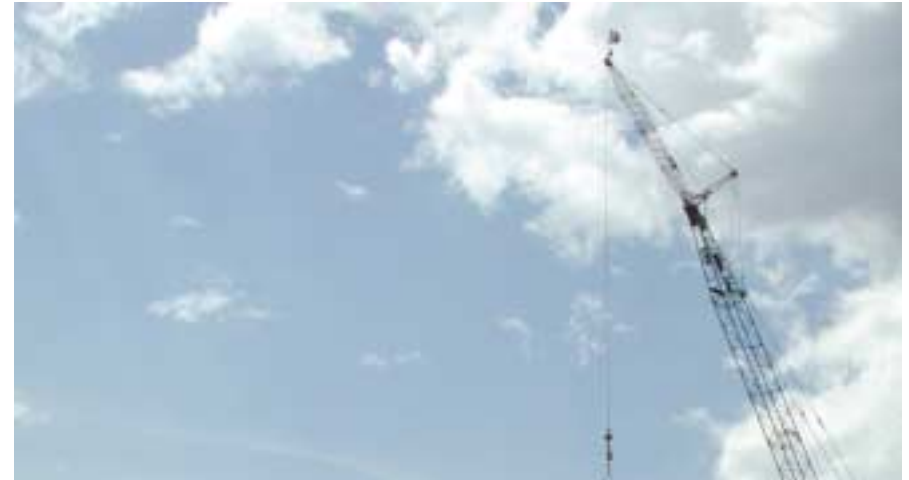
Development continues along the Corridor.
