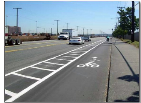
Example of a buffered bike lane in Seattle
