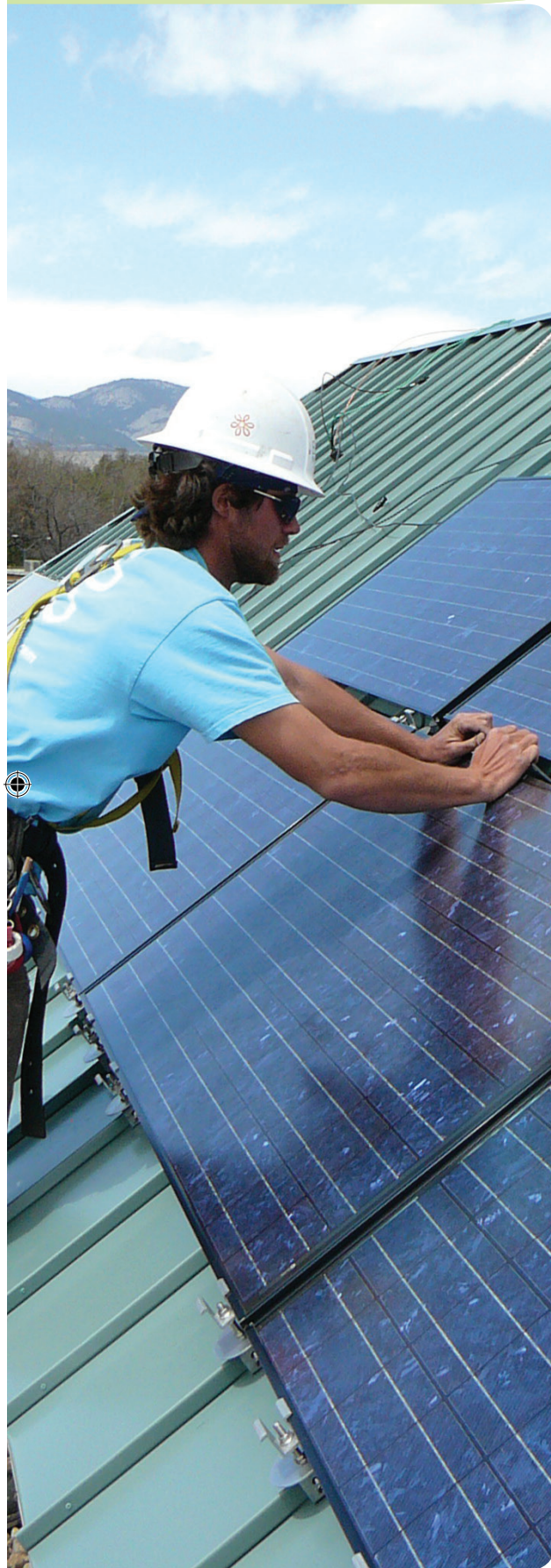
PV Installation at 215 N. Mason St.
