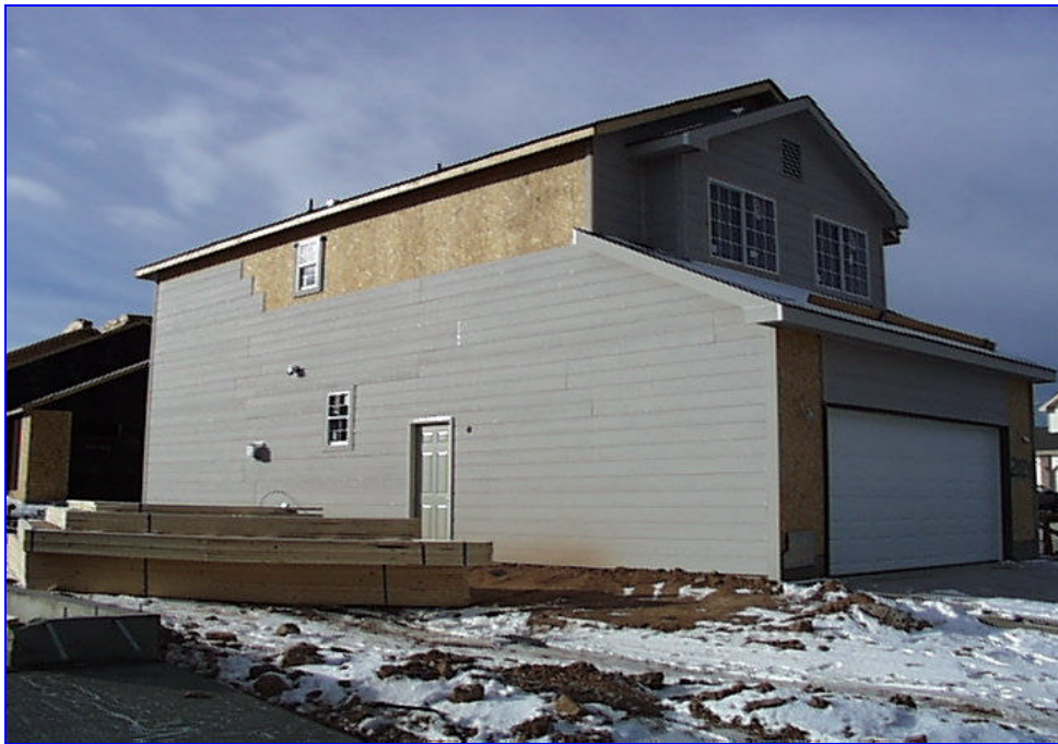
IMAGE 5 – PARTICIPATING BUILDING DURING ‘SIDING’ PHASE.
