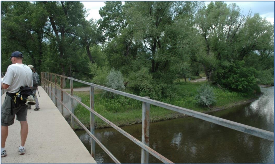
Figure 2.9 McMurry Pedestrian Bridge, Note Non-Compliant Railing
