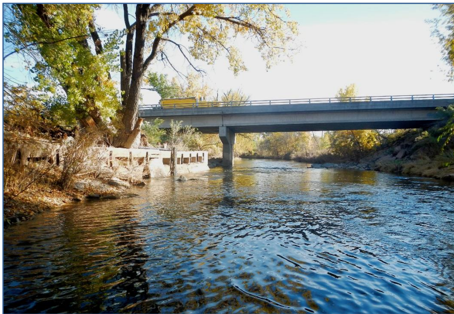
Figure 2.33 Historic Concrete Structure Obstructing the Upstream Side of the Lincoln Avenue Bridge
