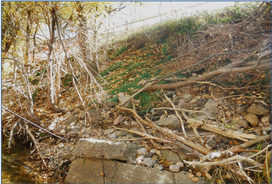
Figure 2.23 Bank Erosion, Concrete Rubble, and Exposed Plastic Turf Mat on South Bank, West of the BNSF Railroad
