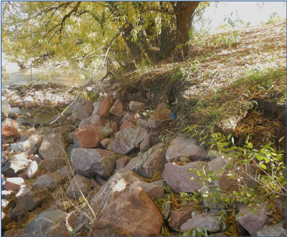
Figure 2.24 Bank Erosion and Exposed Rock Riprap on South Bank, West of the BNSF Railroad
