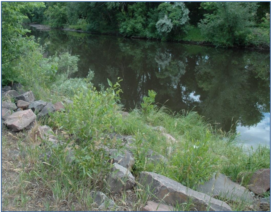
Figure 2.15 Exposed Riprap on the North Bank at Legacy Park
