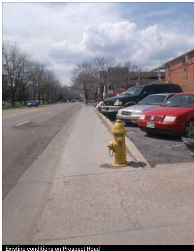
Existing conditions on Prospect Road
