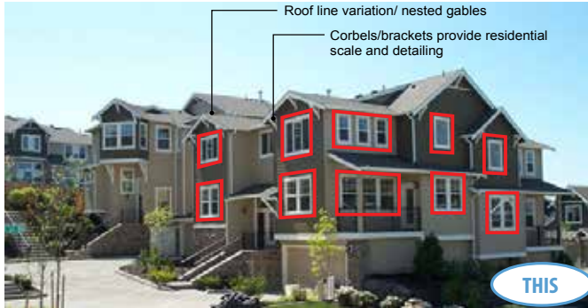
Consistent fenestration and residential detailing
