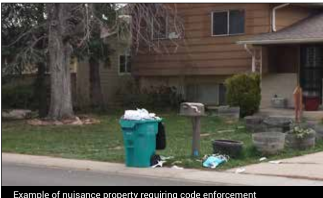
Example of nuisance property requiring code enforcement
