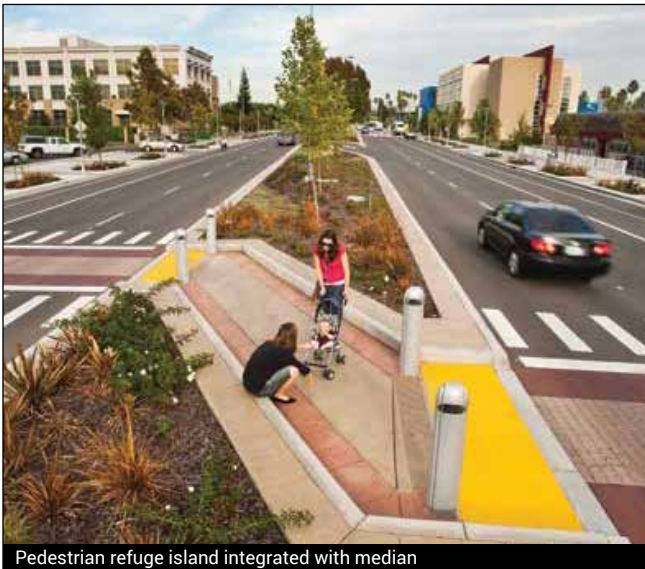
Pedestrian refuge island integrated with median
