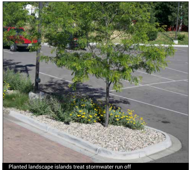
Planted landscape islands treat stormwater run off
