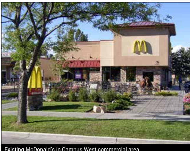
Existing McDonald's in Campus West commercial area
