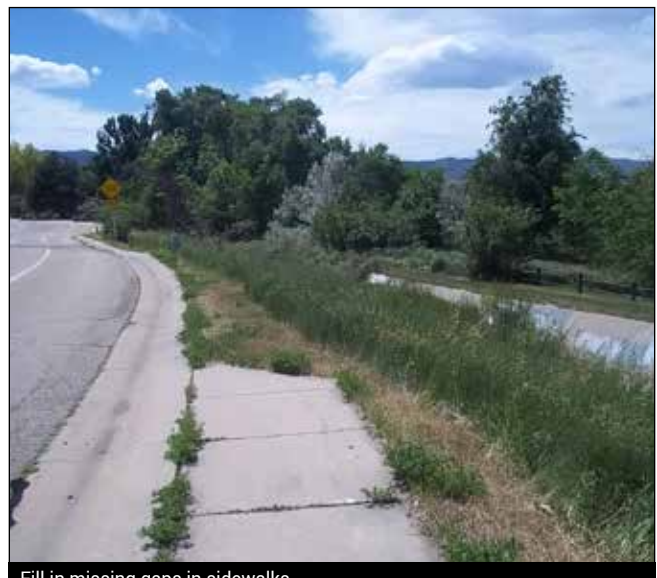
Fill in missing gaps in sidewalks
