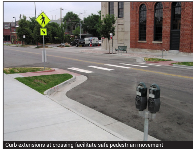
Curb extensions at crossing facilitate safe pedestrian movement
