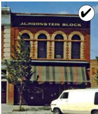
In the early 1980s, the initial rehabilitation revealed key features of the facade.
