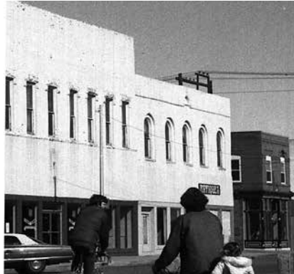
Before rehabilitation (ca. 1980)
