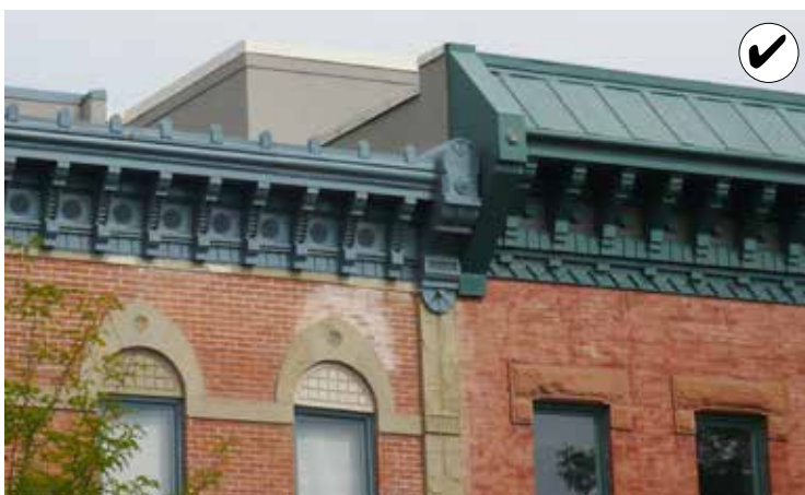
These buildings demonstrate a successful reconstruction of a missing cornice. See the image above for the historic condition. Loomis Building, 213-217 Linden Street
