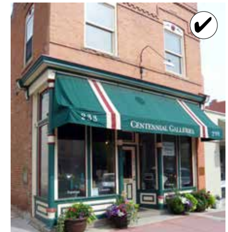
Storefront components continue to be preserved. (2013)
