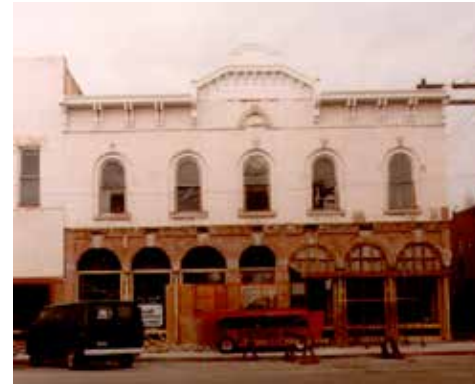
During rehabilitation (ca. 1982)
