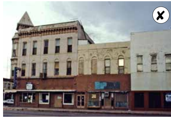
In 1980s, historic masonry is covered with a cementitious plaster and the storefronts have been altered. Some upper story windows have been blocked up.
