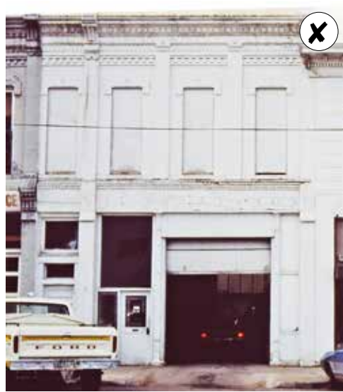
Before rehabilitation: historic windows are missing.
