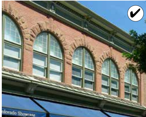
After rehabilitation: repaired windows.
