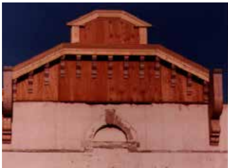
During rehabilitation (ca. 1982)
