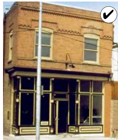
Before rehabilitation: historic storefront components survive. (ca. 1980)
