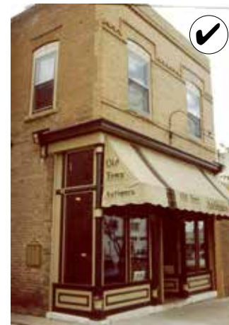
After the initial rehabilitation storefront components are retained. (ca. 1982)
