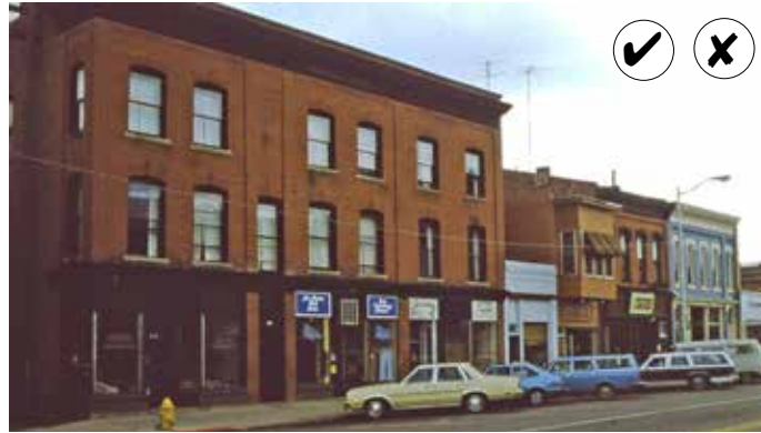
In 1981, many historic features remain, but minor alterations have occurred, and some details are obscured by monochromatic paint schemes.
