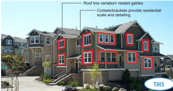
Consistent fenestration and residential detailing
