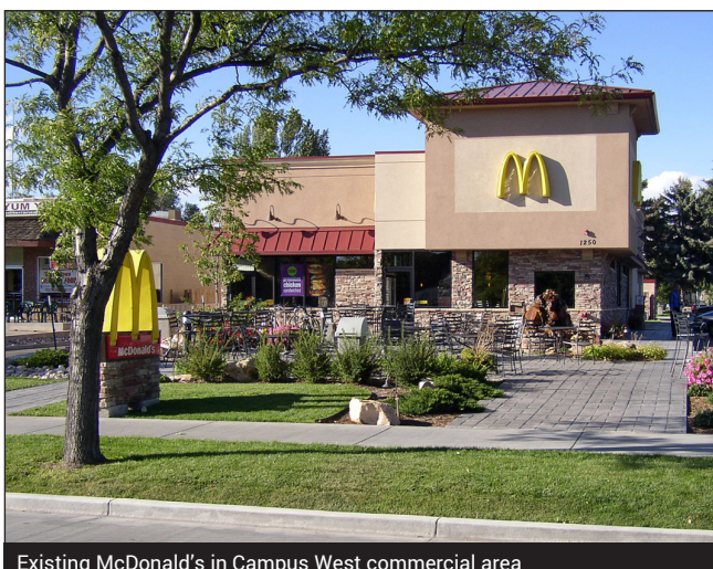
Existing McDonald's in Campus West commercial area
