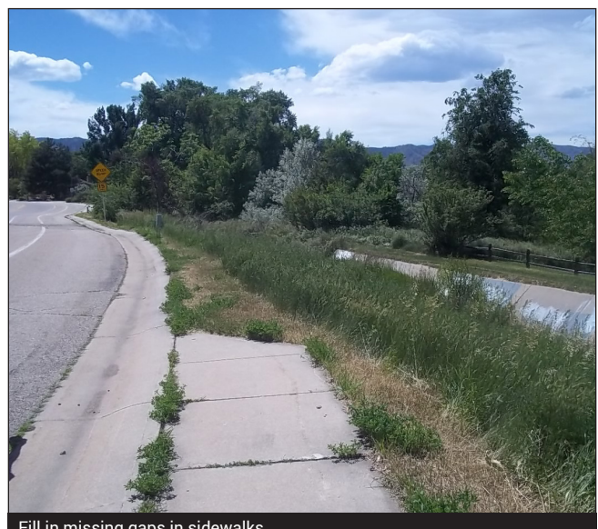
Fill in missing gaps in sidewalks
