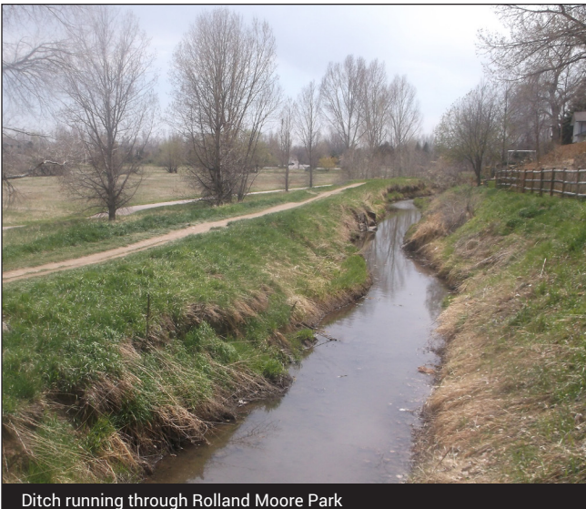
Ditch running through Rolland Moore Park
