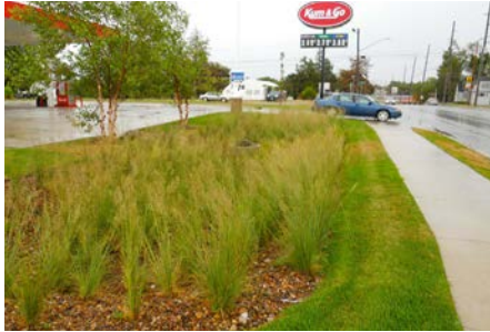
Stormwater Bioswale along Roadway
