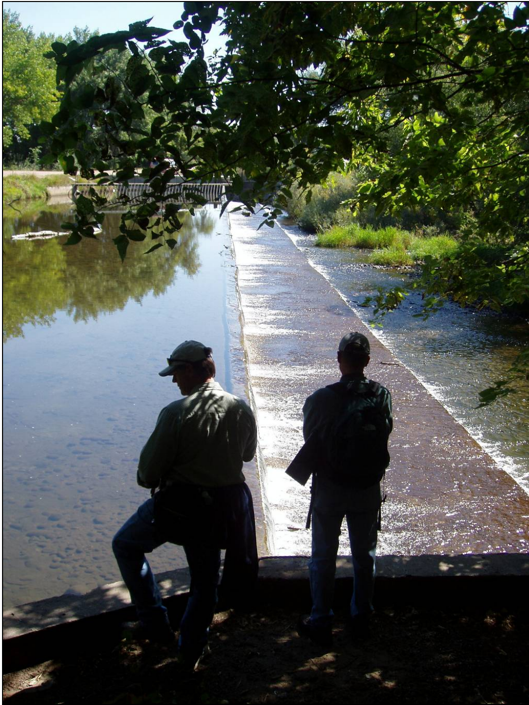
Figure 11. Diversion structure upstream of College Avenue.
