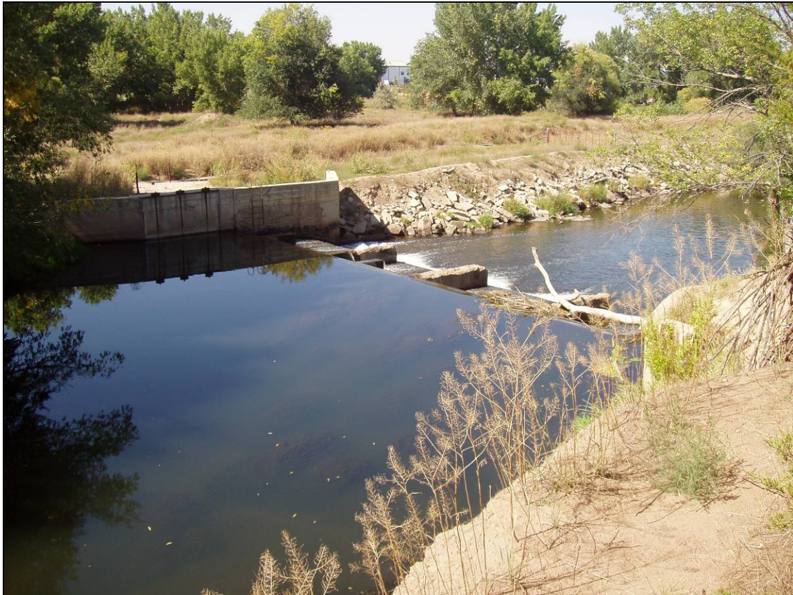
Figure 14. Diversion downstream of Lemay Avenue.
