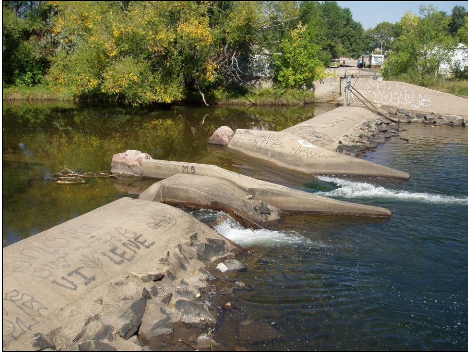
Figure 12. Reconstructed boat chute and fish passage downstream of College Avenue.
