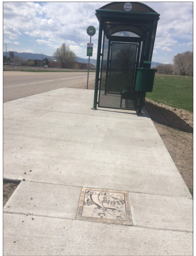
12. Paver at new sidewalk leading to bus shelter at Vine Drive and Alta Vista
