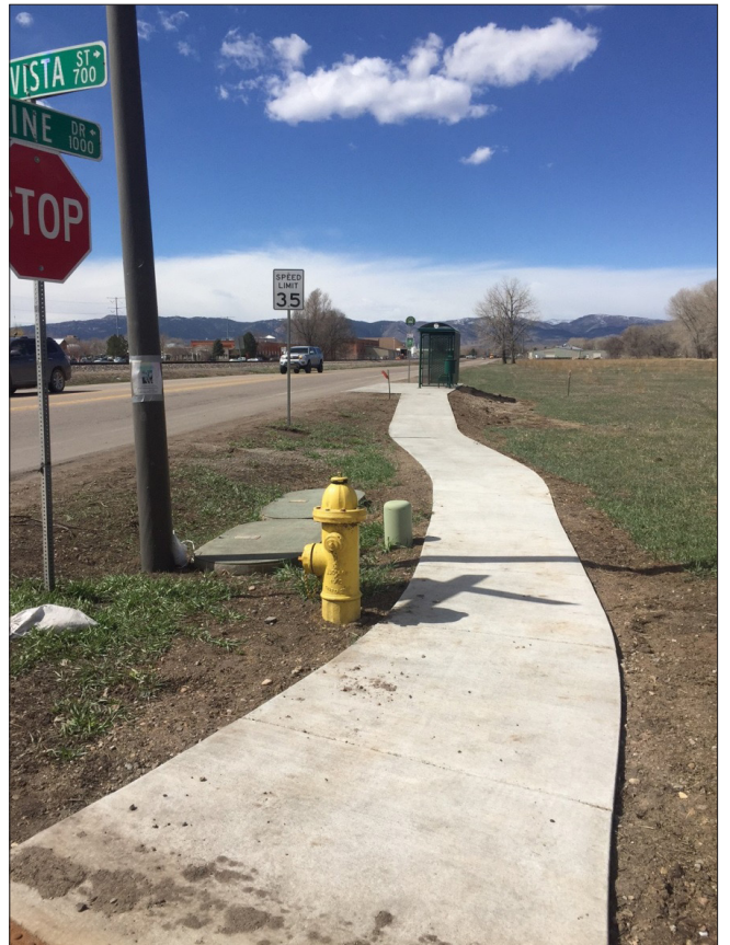
13. Sidewalk leading to bus shelter at Vine Drive and Alta Vista
