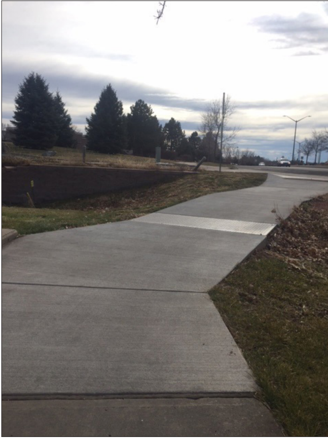
1. Lemay Avenue sidewalk connection south of Buffalo Run Apartments
