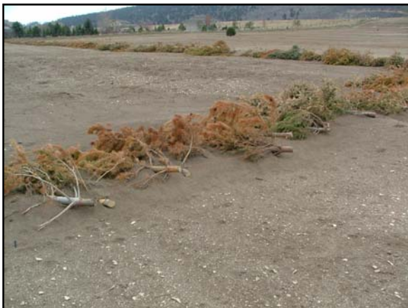
Pineridge Natural Area 2006 (notice Christmas trees were used to capture eroding soils)
