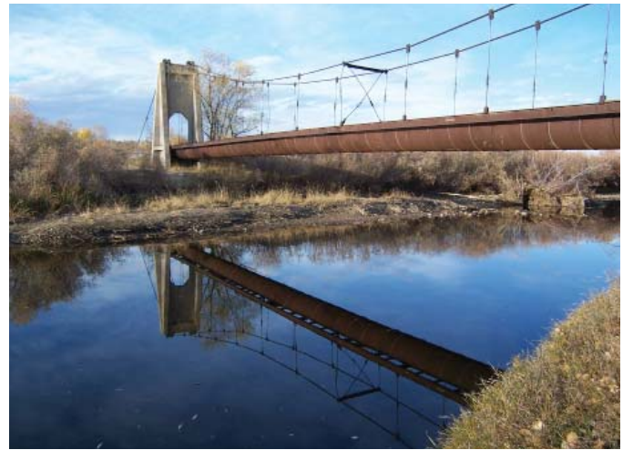
Great Western Sugar Company Beet Effluent Bridge on Kingfisher Point Natural Area (City of Fort Collins Natural Areas Department Photo)
