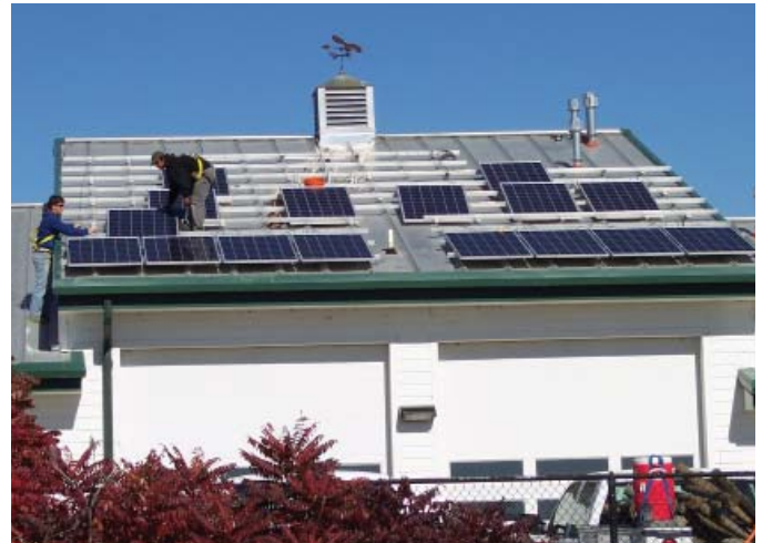
Installation of solar panels on Nix Farm Maintenance Shop (City of Fort Collins Natural Areas Department Photo)
