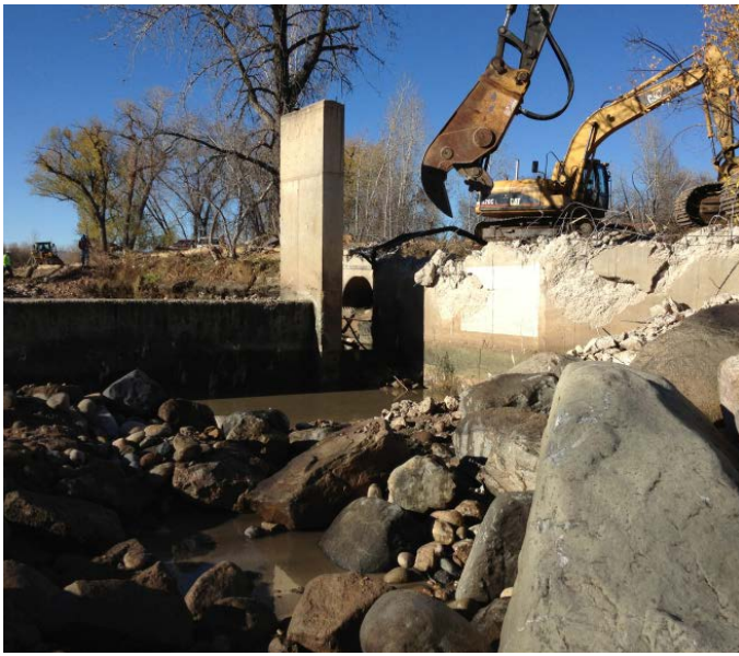
Removal of the Josh Ames Ditch diversion structure at North Shields Ponds Natural Area (City of Fort Collins Natural Areas Department Photo)
