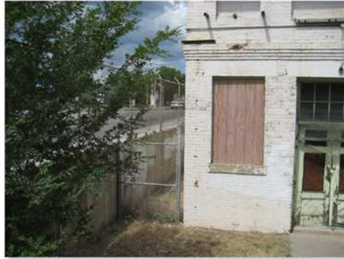
Existing PSCO Building looking southwest along Prospect
