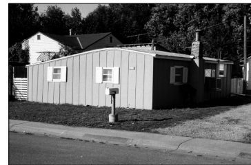
Barrel-roofed hall-and-parlor sugar beet shanty with a shed-roof addition to the south elevation (left), located at 209 Third Street in Buckingham.
