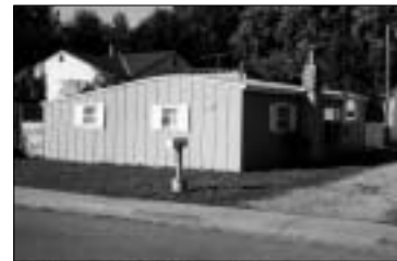
Barrel-roofed hall-and-parlor sugar beet shanty with a shed-roof addition to the south elevation (left), located at 209 Third Street in Buckingham.
