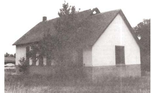
Figure 30. The Fossil Creek School before its demolition in 1986. (Photo by Marilyn Norlin Eckles, in Morris , vol. II)
