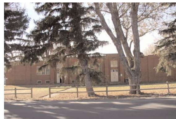
Figure 35. The Waverly School was a rather sophisticated and large building for its rural location. (Photo by the author)
