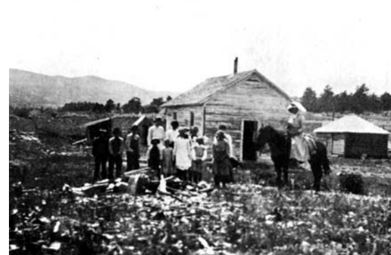
Figure 38. The Westlake School, photographed in 1912. The small building at right is a horse shelter. (Swanson, Red Feather Lakes)
