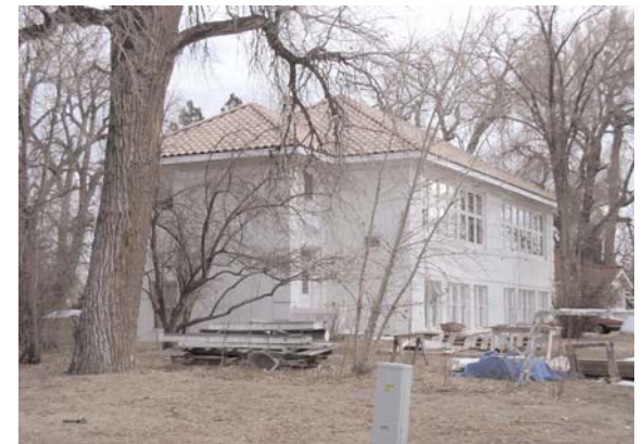
Figure 23. Located on the north side of Highway 14 (Mulberry Street) just east of Interstate 25, the Lower Boxelder School (above) and its matching teacherage are now private residences. (Photo by the author.)
