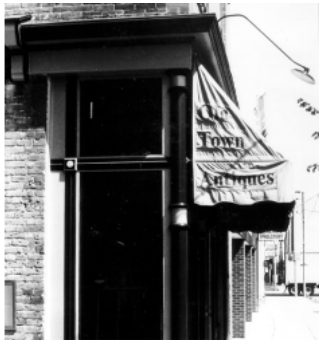
In general, an awning is more successful as a combination sign and weather control device than are horizontal canopies.
