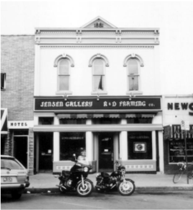
In general, signs should not overpower the image of the facade as a single composition.
