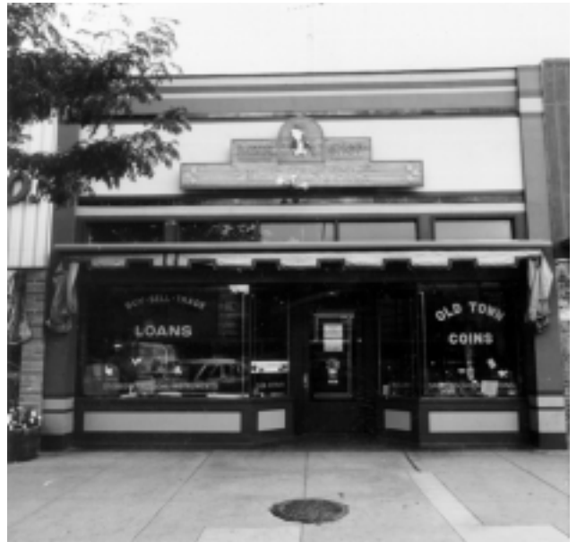
and after - a contemporary modification
