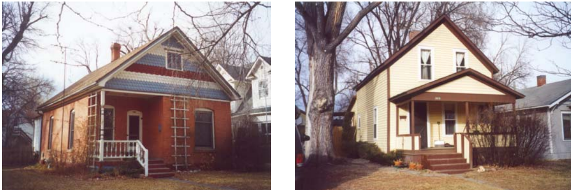
Figure 19. Modern views of two houses relocated from the Old Fort Site in 1910 to make way for the UP Railroad, including 721 Smith Street (left) and 1018 Akin Street (right).
