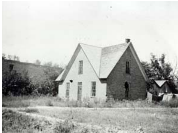
Figure 8. The Peterson house on Lincoln Avenue, reportedly the first brick house erected in Fort Collins (Source: Fort Collins Public Library, Local History Archives).
