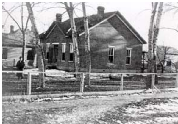
Figure 15. Brick home built by Frank Stover in 1878 on the southeast corner of Linden and Willow Streets (Source: Fort Collins Public Library, Local History Archives).
