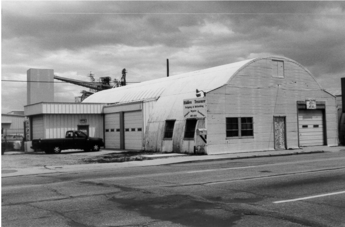
Figure 23. Ex-military Quonset hut placed at 400 Jefferson Street in 1948-49 and occupied initially by the C.G. Richardson Manufacturing Company.
