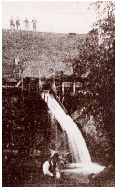
Figure 7. Water from the millrace being discharged back into the Poudre River via a wooden flume at the Peterson and Stone grist mill (Source: Watrous 1911).
