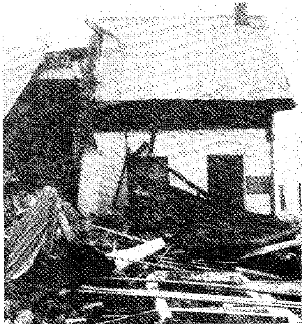
Demolition of Rhodes House
