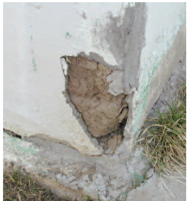
Figure 6. Adobe bricks show through a crack in the stucco of this Alta Vista house. (Photo by the author.)
