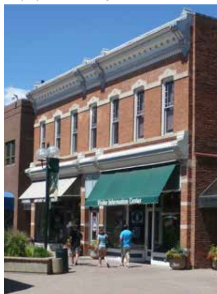
Ca. 1980, Black's Glass, with a missing mid-belt molding, and historic storefront altered. The transom also is covered, changing the proportions of the ground level.
