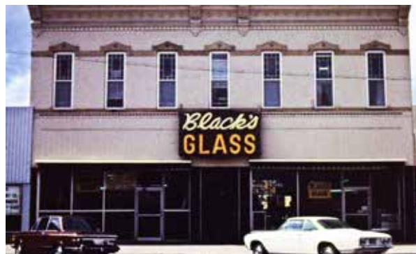
Ca. 1980, Black's Glass, with a missing mid-belt molding, and historic storefront altered. The transom also is covered, changing the proportions of the ground level.
