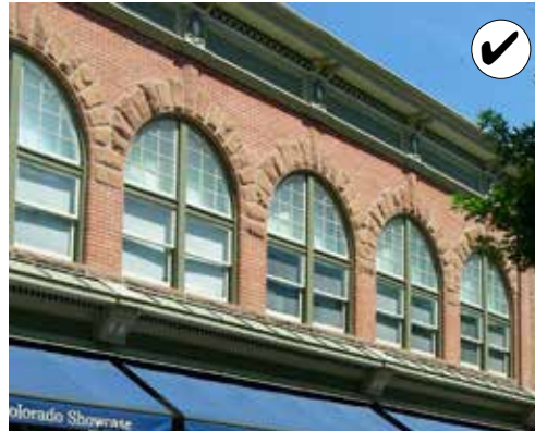
After rehabilitation: repaired windows.
