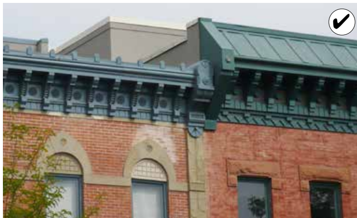
These buildings demonstrate a successful reconstruction of a missing cornice. See the image above for the historic condition.
