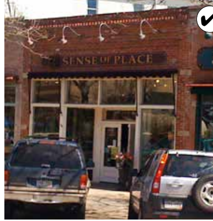
A later rehabilitation effort included removing the stucco, reconstructing the cornice and installing a new storefront system.
