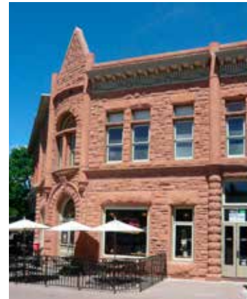
In 2013, a reconstructed cornice reestablished a distinctive horizontal feature, and awning once more reflect the dimensions of each storefront bay.
