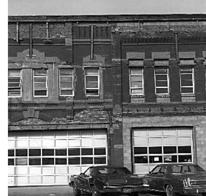
At the beginning of rehabilitation in the early 1980s, damage to the historic masonry is visible. The hose tower also is missing.
