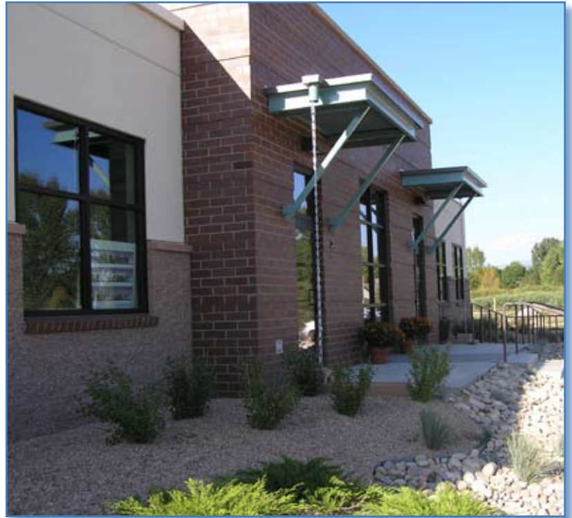
Careful window selection provides daylighting and views while minimizing unwanted heat gain.
