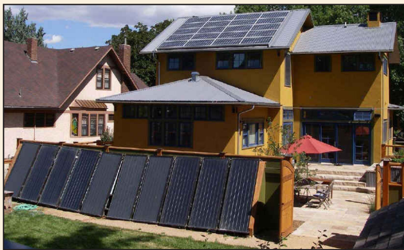
Fort Collins Zero Energy Home
