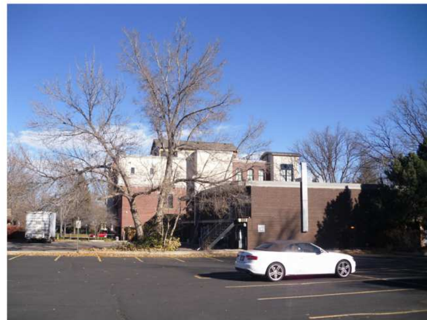
VIEW OF EXISTING BUILDING LOOKING AT THE SOUTH ELEVATION
