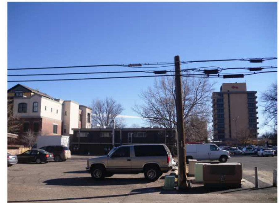
VIEW OF EXISTING BUILDING LOOKING AT THE WEST ELEVATION
