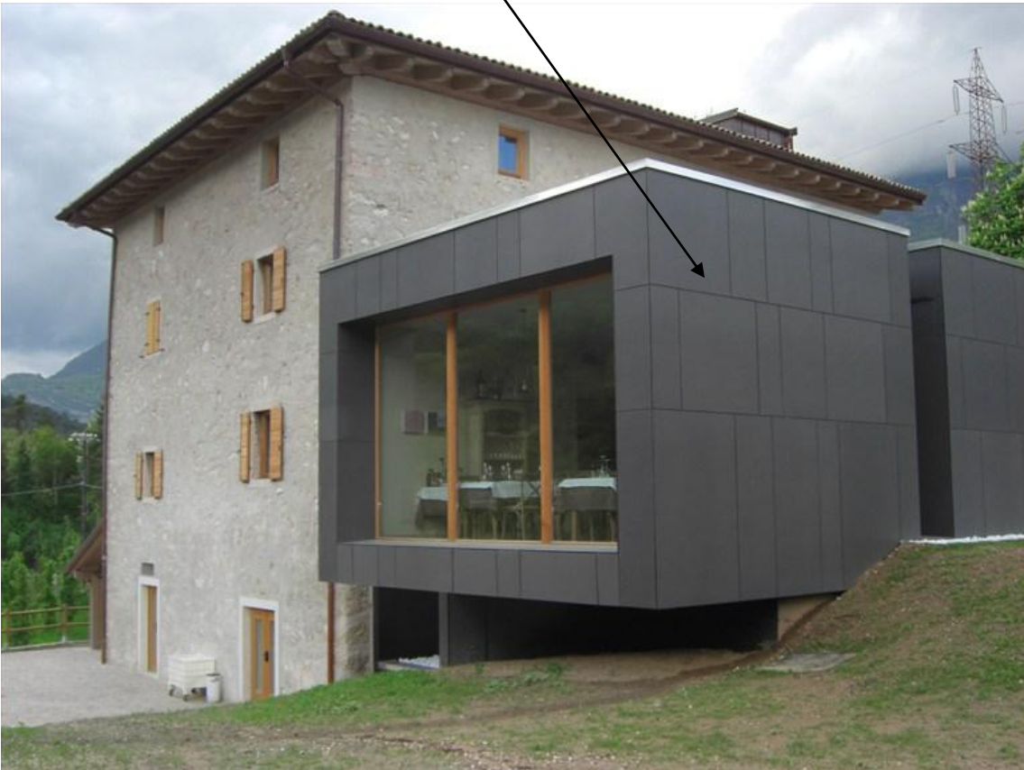
Image of installed Swiss Pearl (dark grey panel)
