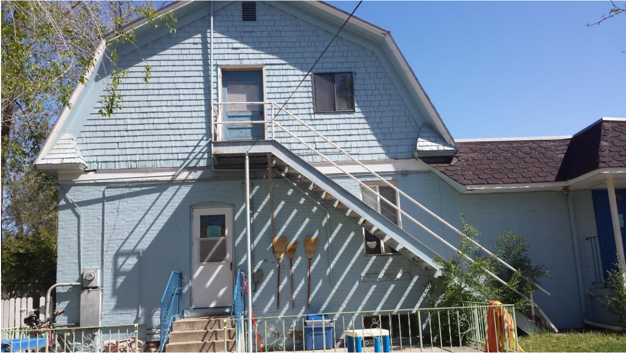
Back of Building
