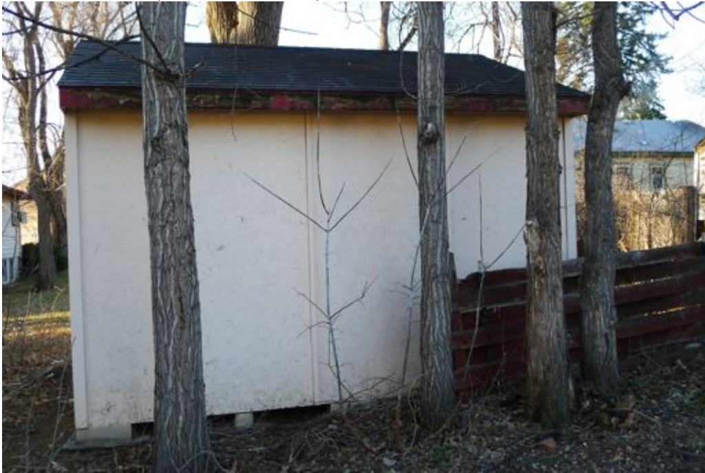
Shed northern wall (taken from alleyway), photo faces south
