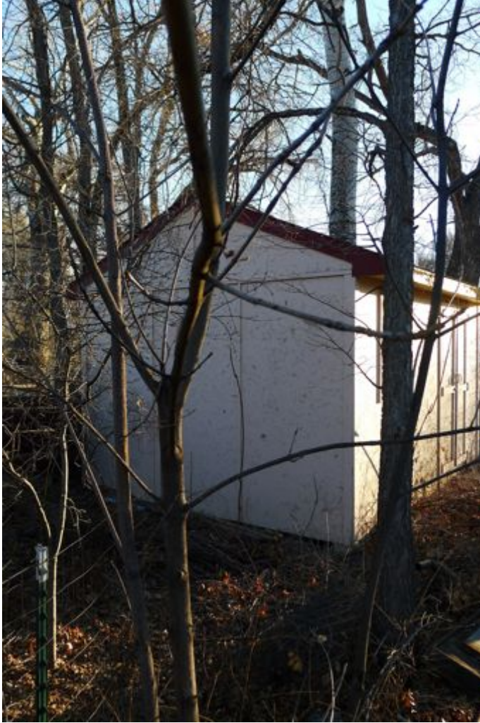
Shed western wall, photo faces east
