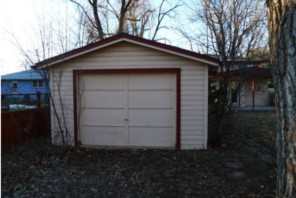
Garage northern wall (taken from alleyway), photo faces south
