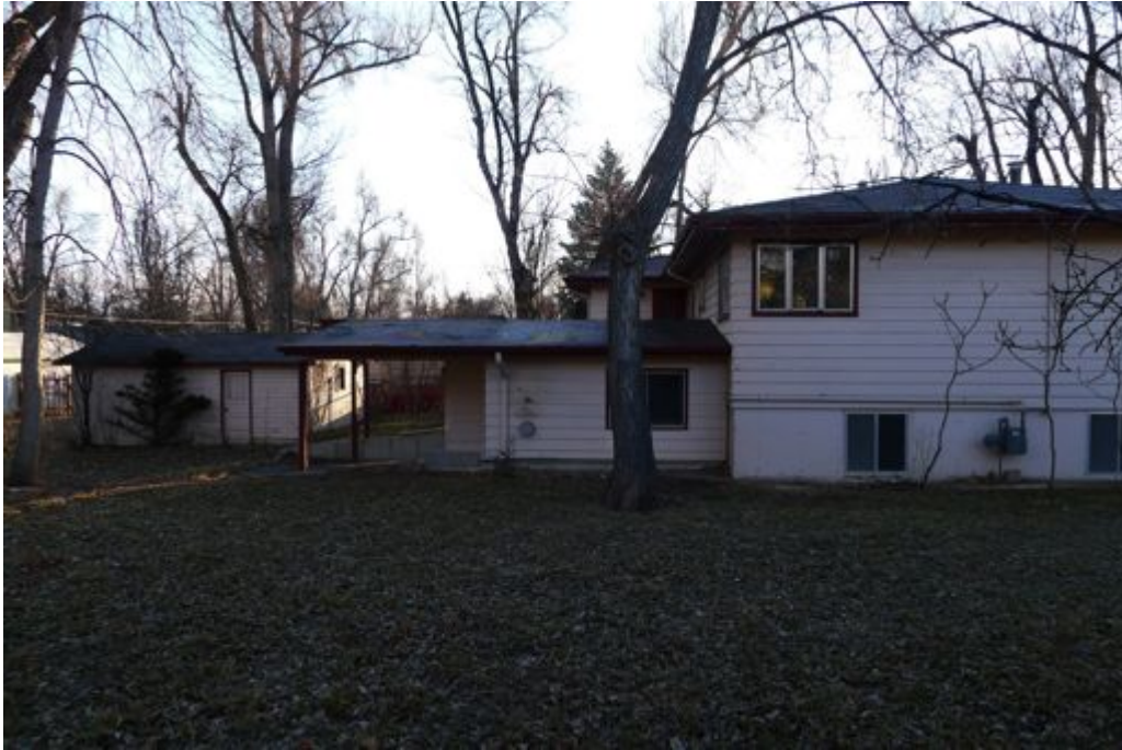
House western wall, photo faces east
