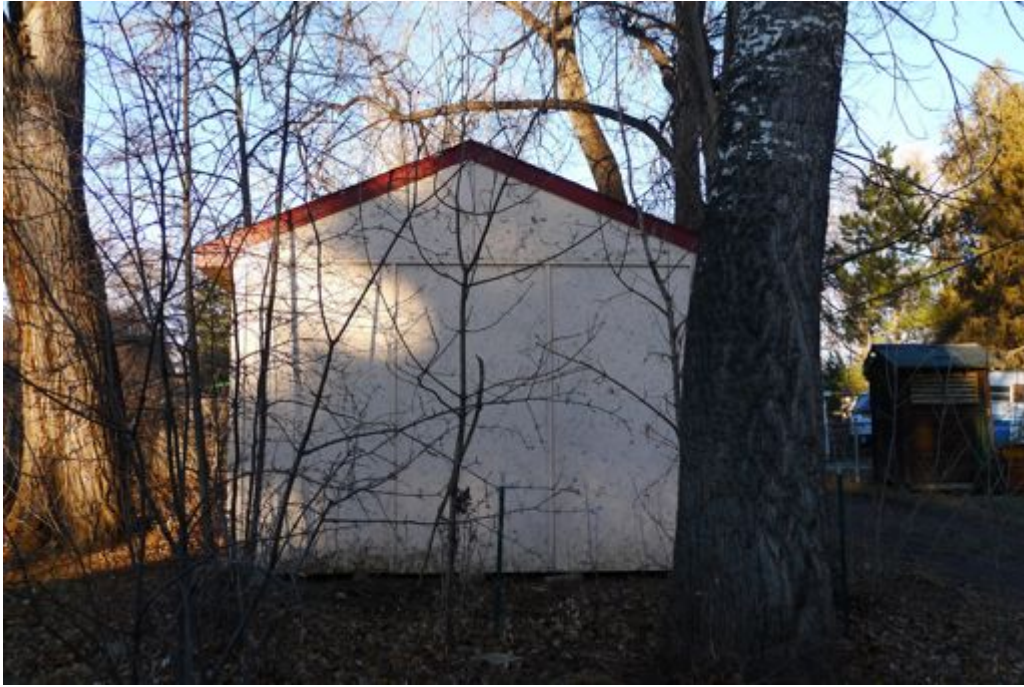
Shed eastern wall, photo faces west
