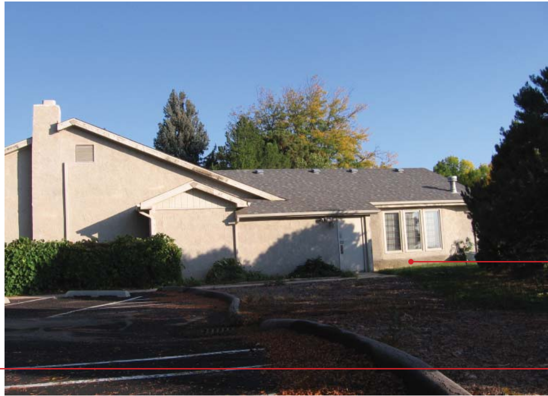
SOUTH SIDE OF EXISTING EVENT STRUCTURE
