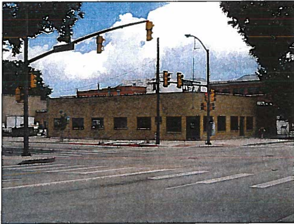
Lane Foundry Building. West & south elevations. View to the northeast.
