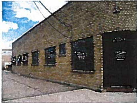
Southwest Building Corner
