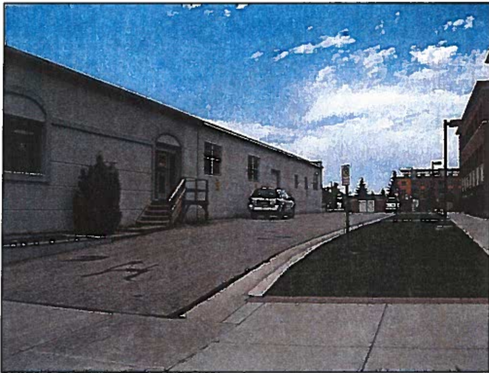
East elevation. View to the northwest.
