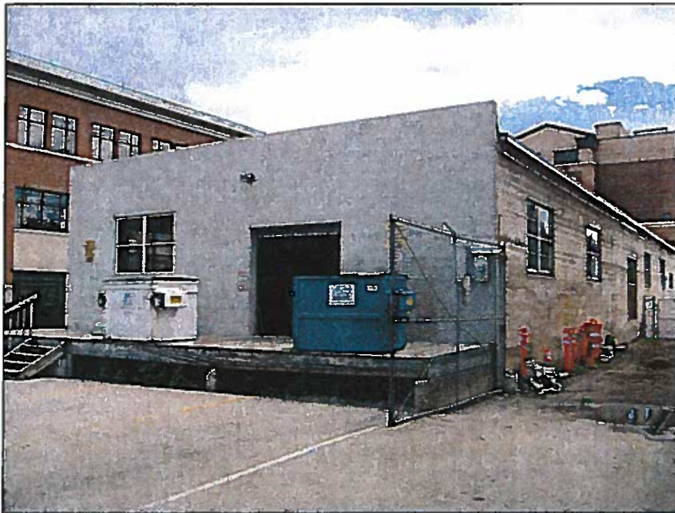
Rear of the Building. North & west elevations. View to the southeast.
