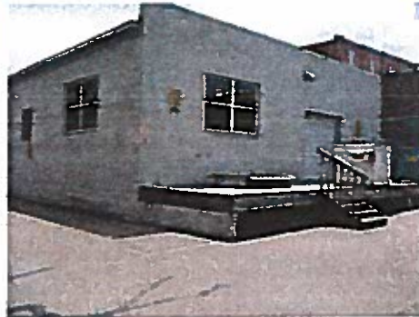
Northeast Building Corner
