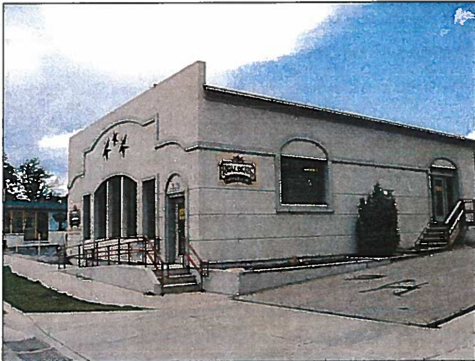
South & east elevations. View to the northwest.
