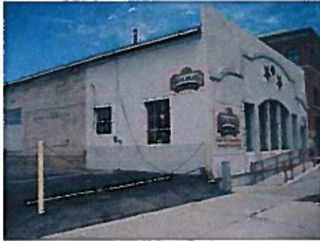
Southwest Building Corner
