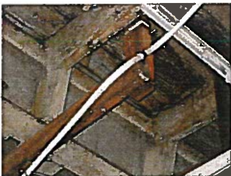
Rafters to Steel Beam Connections (East Side of Building)
