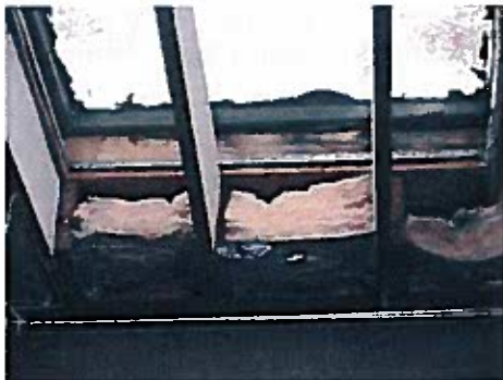
Water Damage at Skylight
