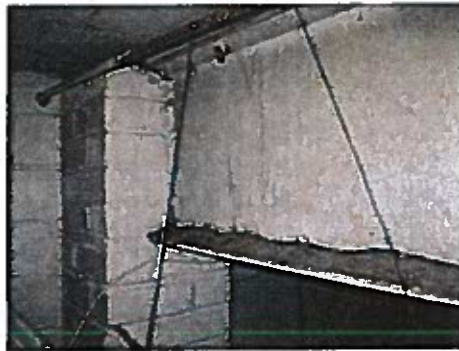
Northern-most Steel Beam Line (West Side of Building)
