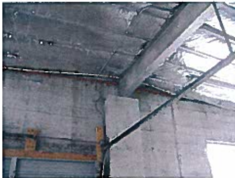
Steel Beam and Concrete Pilaster (North Wall of Building)
