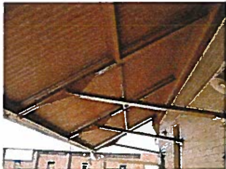
Steel Angle Trusses at Overhang
