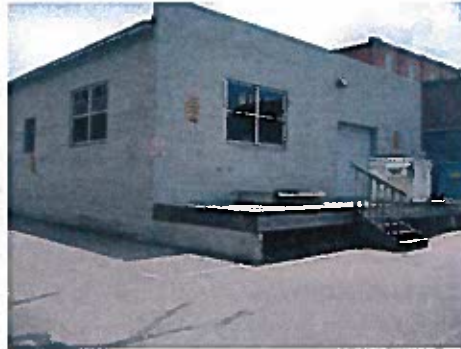
Northeast Building Corner
