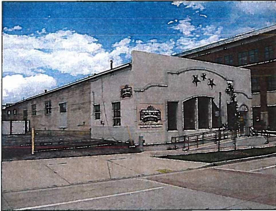
Hanna Turkey Store Building. West & south elevations. View to the northeast.
