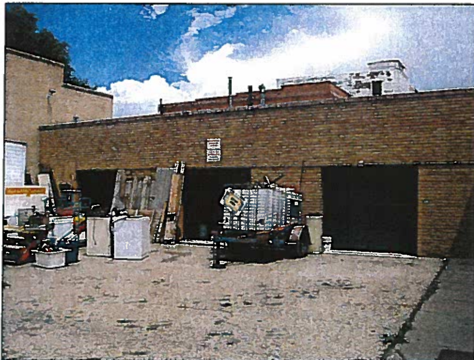
North Addition. West elevation. View to the northeast.
