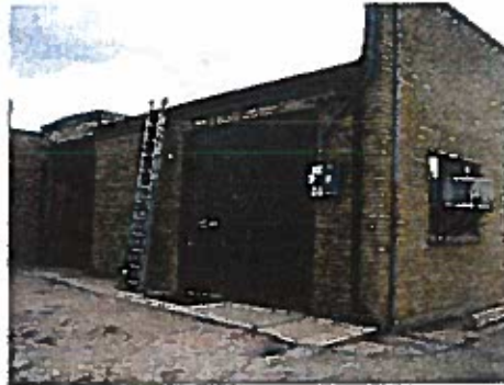
Northwest Building Corner
