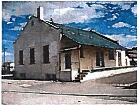
Northwest Building Corner
