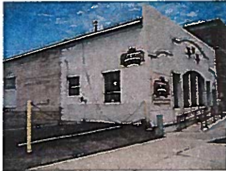
Southwest Building Corner
