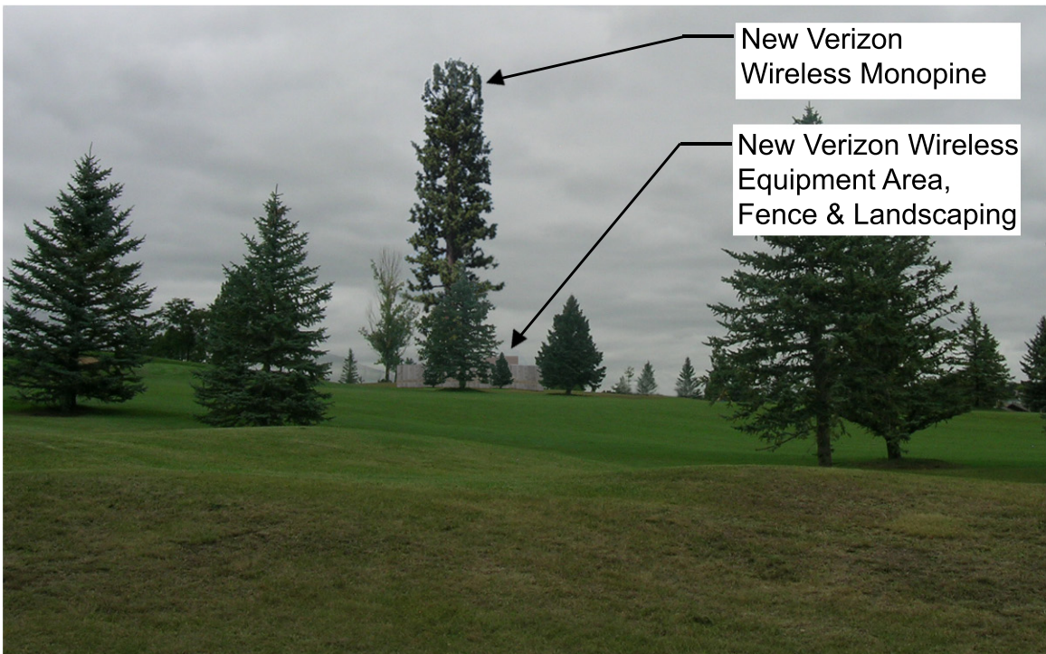
New Verizon Wireless Monopine w/ Antennas & Equipment Area
