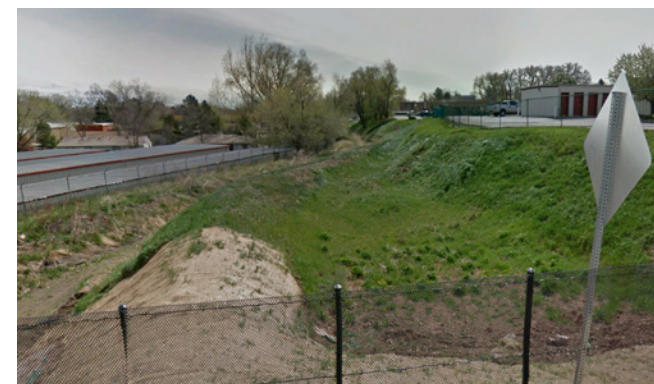
EXISTING DETENTION POND AND 1.5:1 SLOPE
