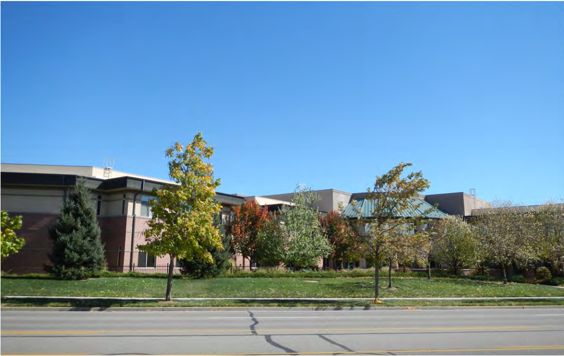
Existing View from the Northwest
