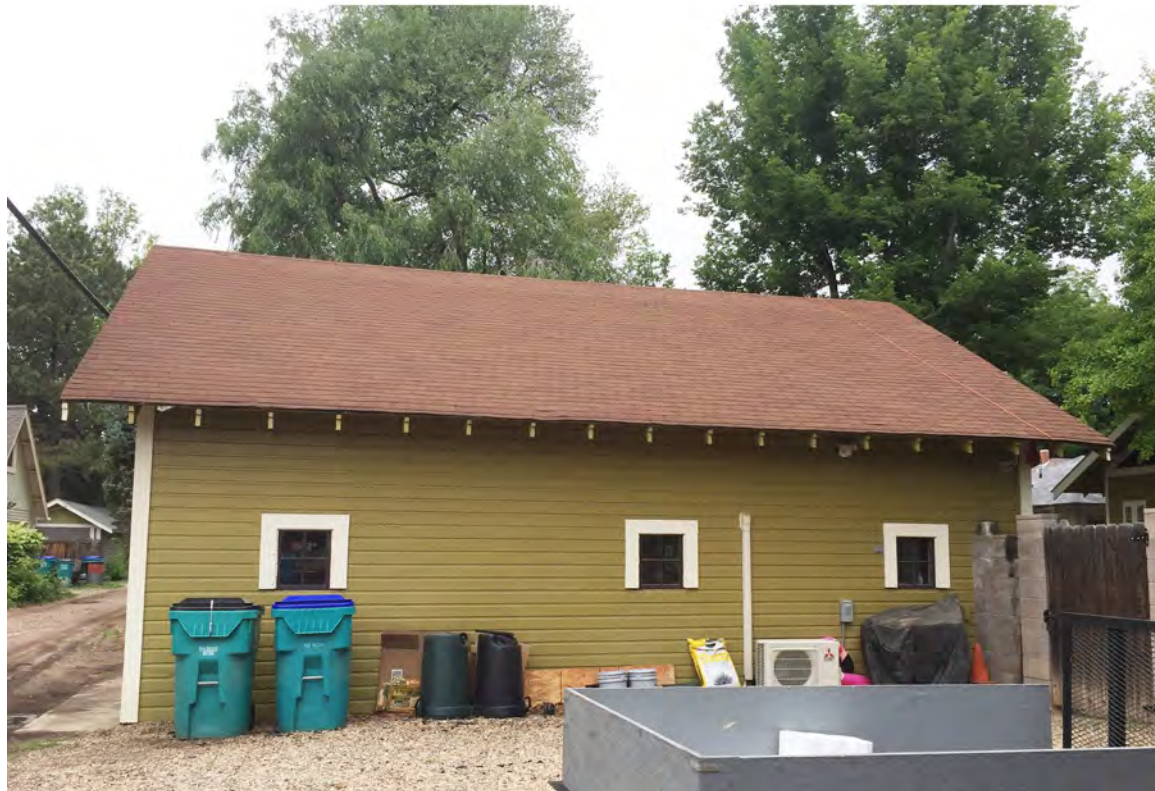
1115 W. Mountain Avenue Garage East Elevation
