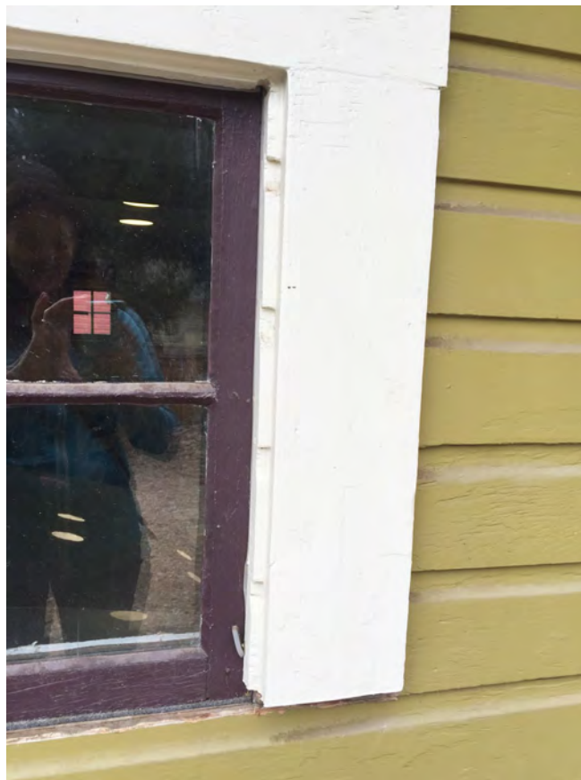
1115 W. Mountain Avenue Garage Typical Window
