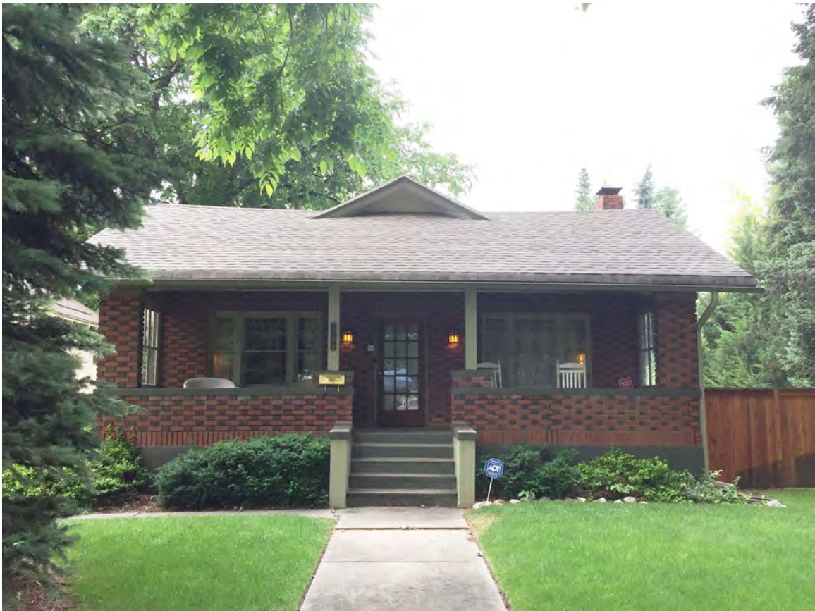
1105 W. Mountain Avenue North (street) Elevation
