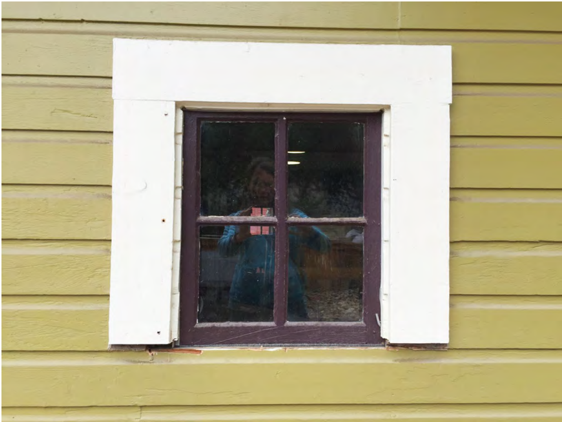
1115 W. Mountain Avenue Garage Typical Window
