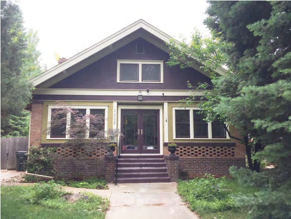
1115 W. Mountain Avenue North (street) Elevation
