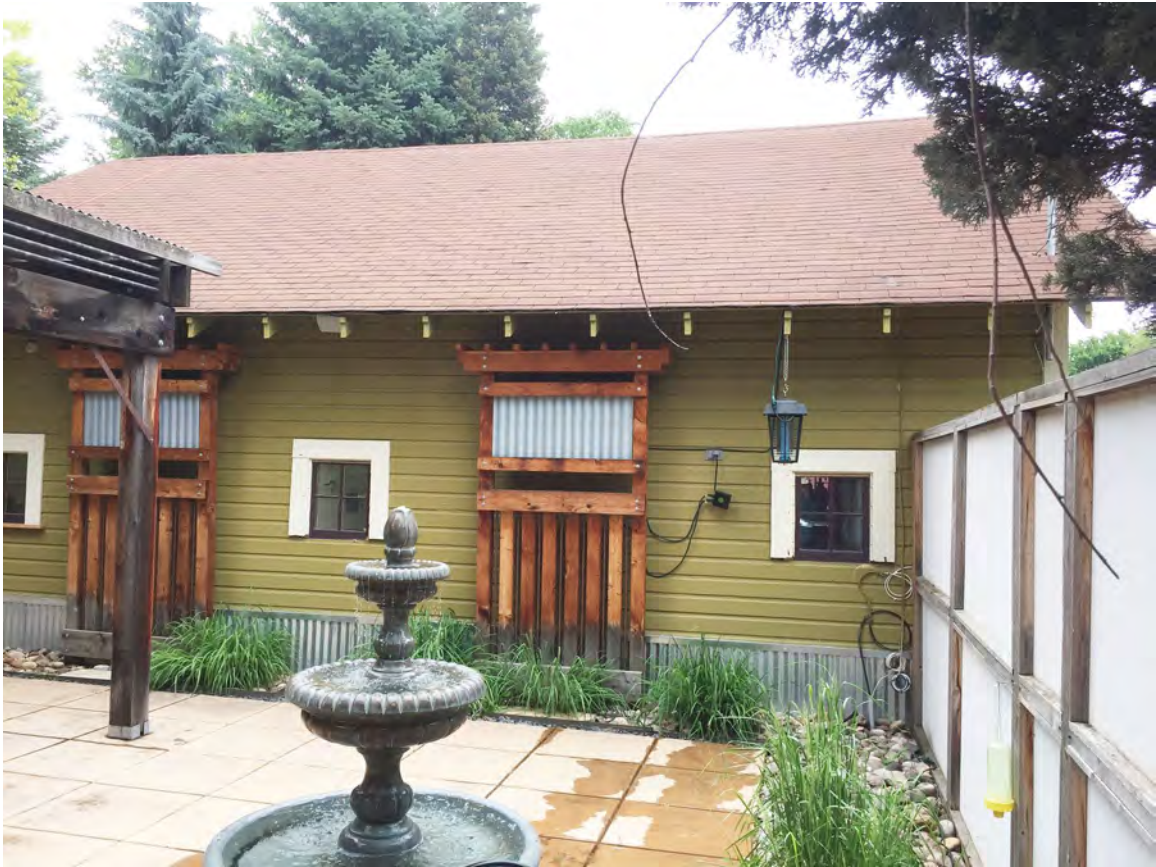
1115 W. Mountain Avenue Garage West Elevation
