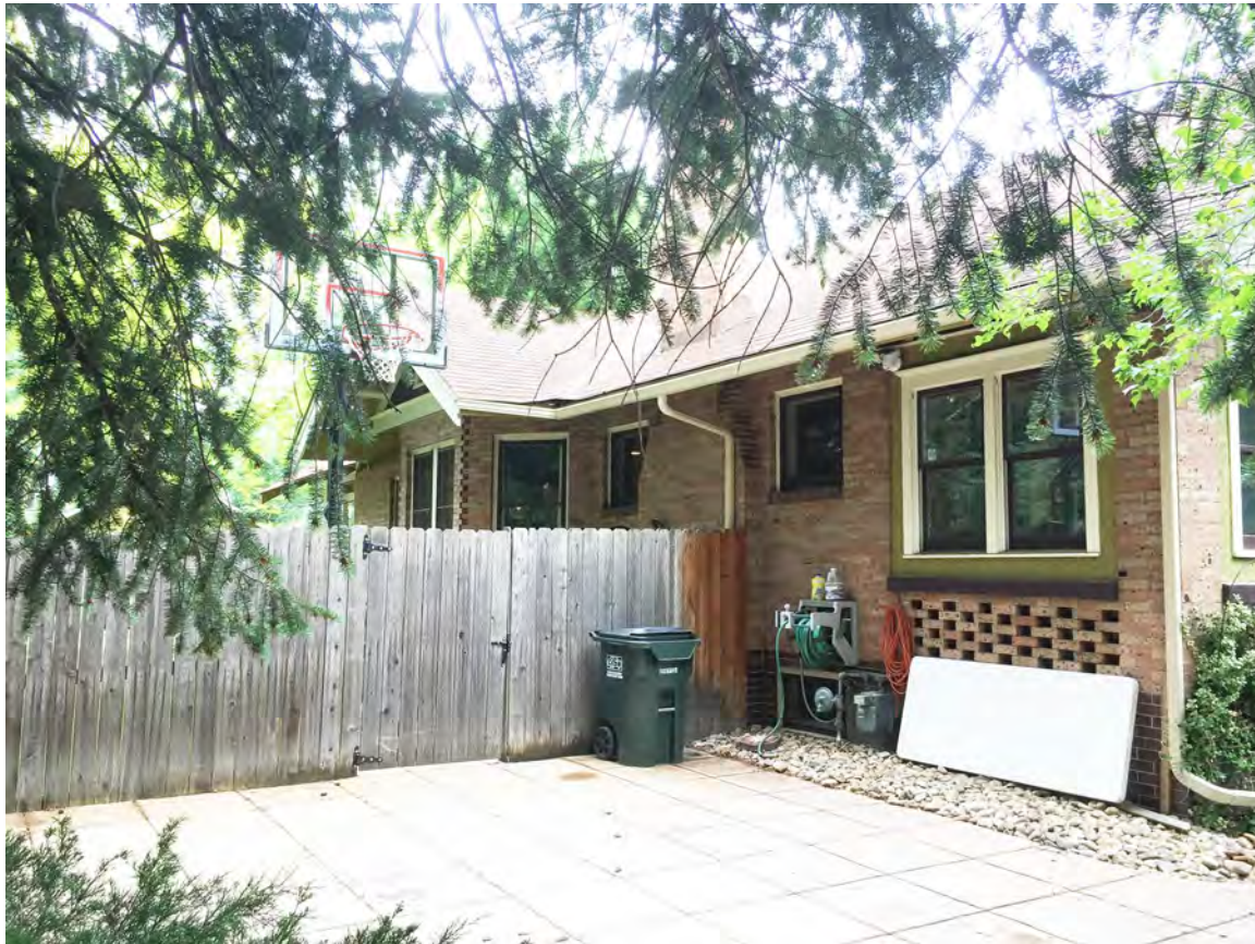
1115 W. Mountain Avenue Northeast Elevation
