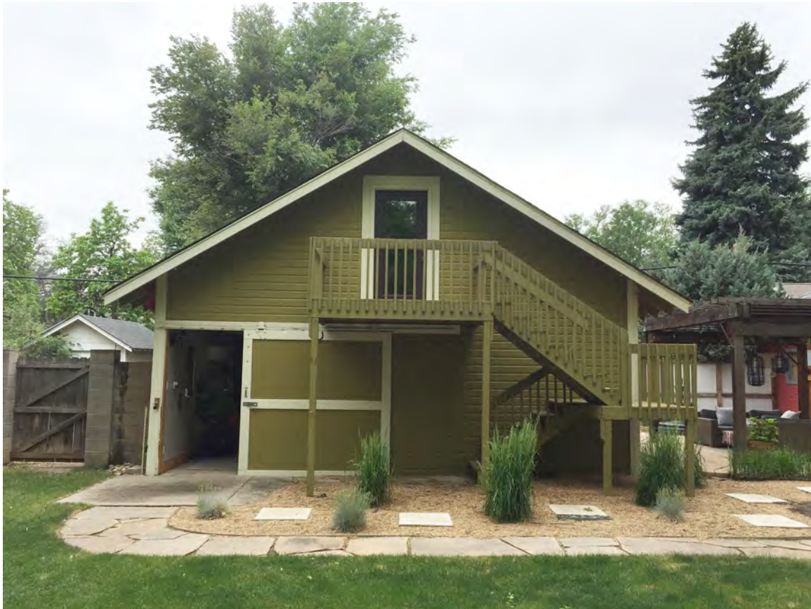
1115 W. Mountain Avenue Garage North Elevation
