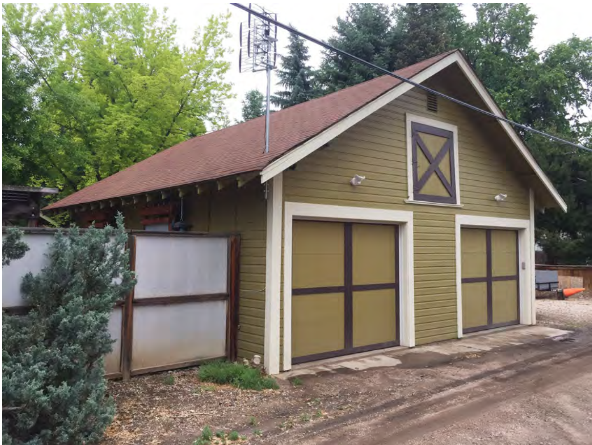
1115 W. Mountain Avenue Garage Southwest Elevation
