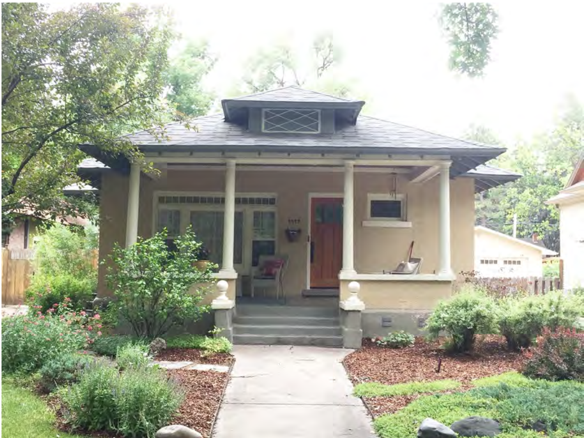
1119 W. Mountain Avenue North (street) Elevation
