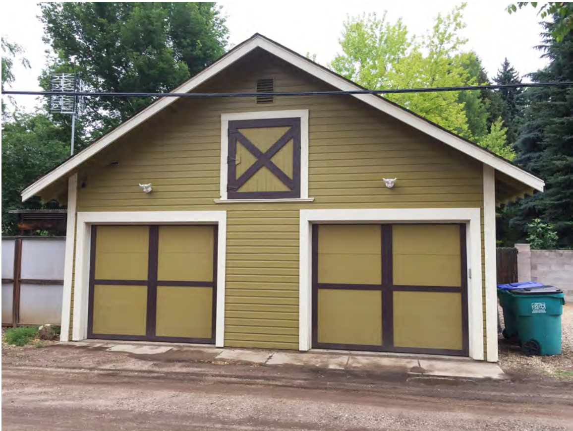
1115 W. Mountain Avenue Garage South Elevation
