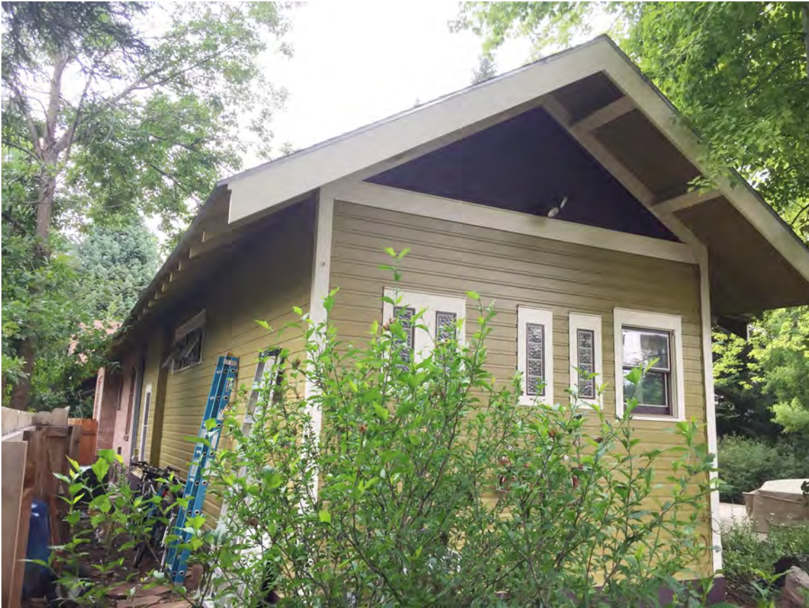
1115 W. Mountain Avenue Southwest Elevation
